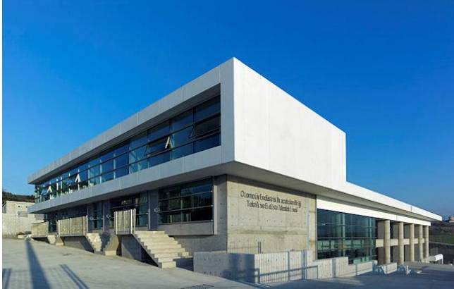
Figure A14 Turkey’s First and only Educational and Public Building with BREEAM “very good” Certificate
