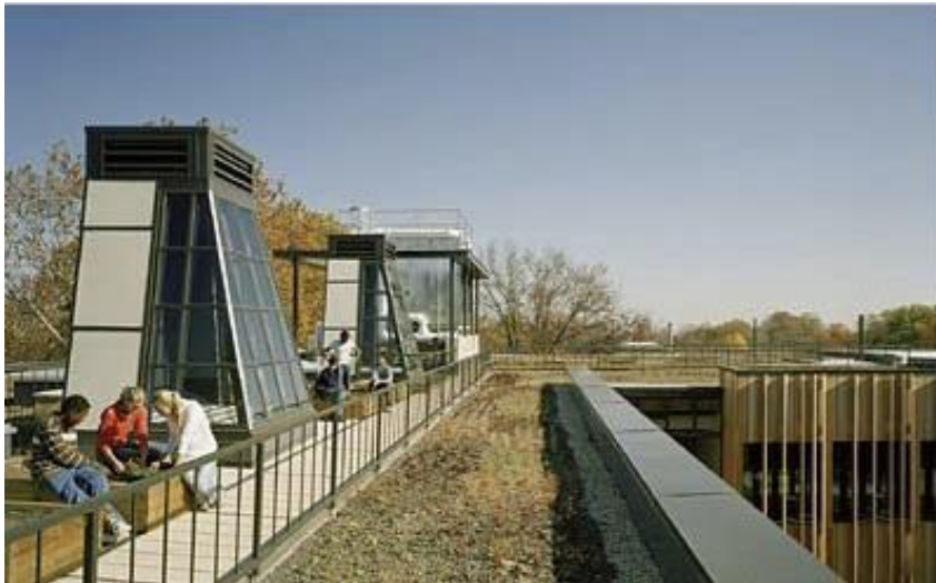
Figure A25 Solar chimney ventilation (LPA, 2009)
