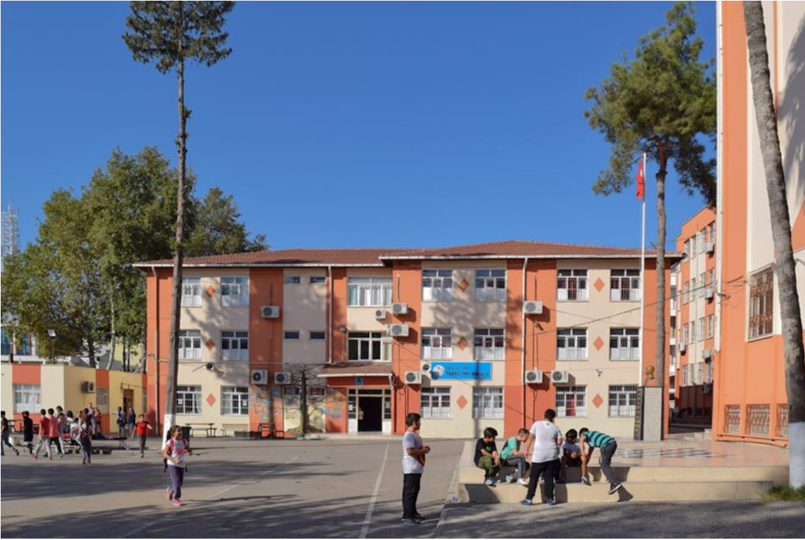
Figure 3.2 The general view of examined secondary school building
