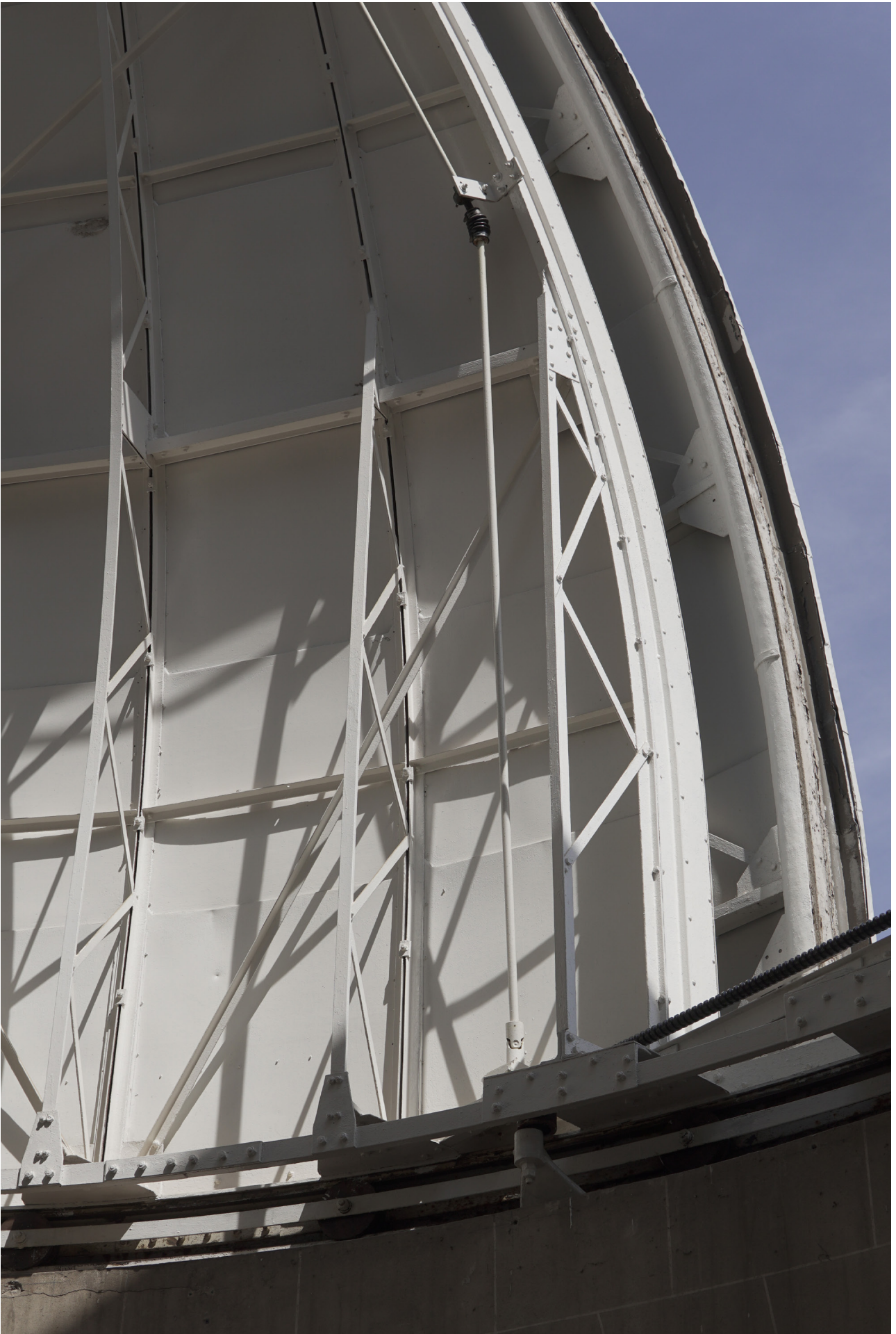
Eiffel's dome detail, Meudon Observatory, 2020.
