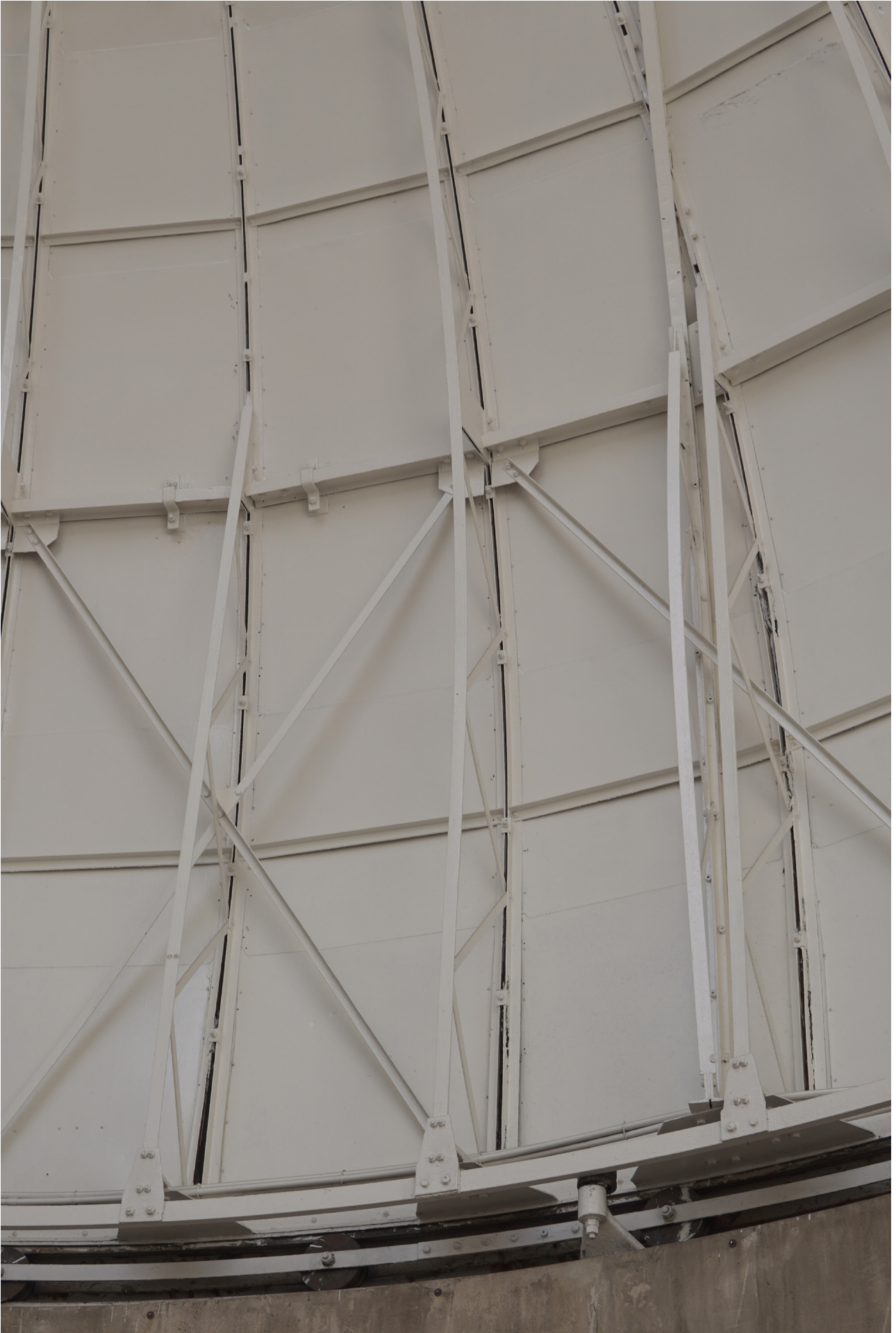
Eiffel's dome detail, Meudon Observatory, 2020.
