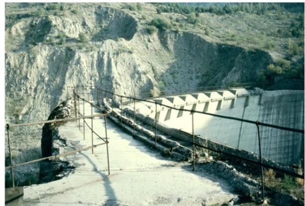
**Fig. 13** View across the top of the dam showing the remains of the road in the foreground (right side of the dam) and the missing parapet wall at the far right of the photo (left side of the dam). Photo: ENB.
