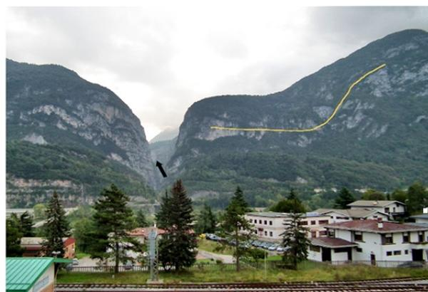
**Fig. 5** The left abutment of the dam (indicated by the black arrow) as seen from a hotel breakfast table in Longarone. One bedding plane is highlighted in yellow to show the 'chair'-shaped structure visible in the cliff at the south side of the gorge. Photo: APD.
