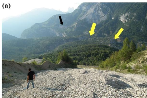
**Fig. 12** (a) View downstream (to the west) across the landslide from high up the east side failure scar. The yellow arrows indicate the leading edge of the failed mass above the northern side of the gorge, and the black arrow indicates Casso village. (b) View past the dam (lower left) from the left side towards Casso (indicated by black arrows). The main part of the village is behind and above the top of the cliff (out of sight) at the lower arrow. Photos: APD; ENB.
