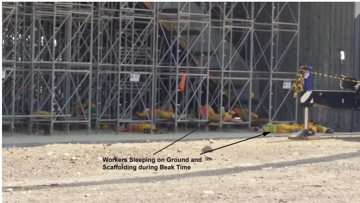
Figure 6: Workers Taking Rest During Break Time on Ground and Scaffolding.
