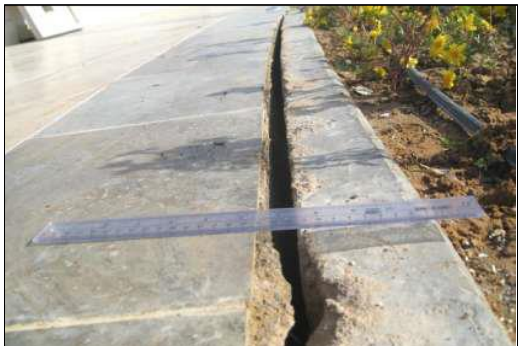
Figure 3.2 Separation of edge kerbstones due to settlement of adjacent green area
