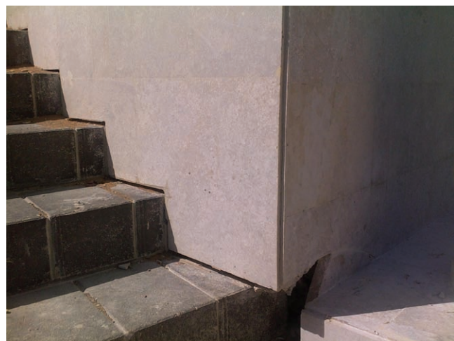
Figure 3. Separation of stairs from adjacent wall due to differential settlement
