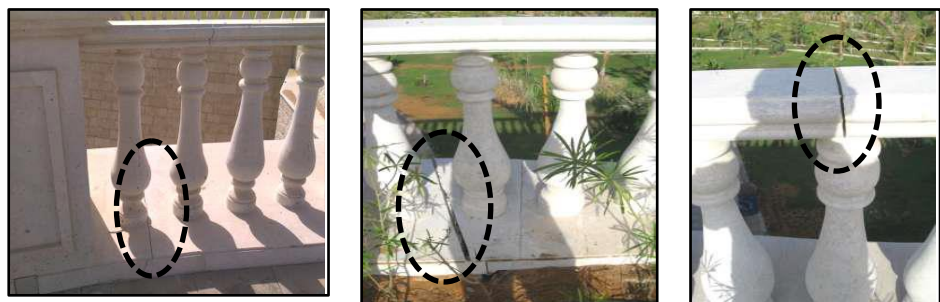
a) Cracking in coping b) Opening of joints c) Crack in rails
