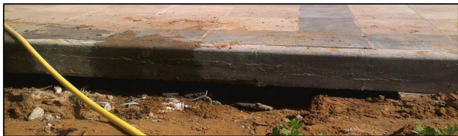
Figure 3.4 Ground subsidence beneath pavement slab
