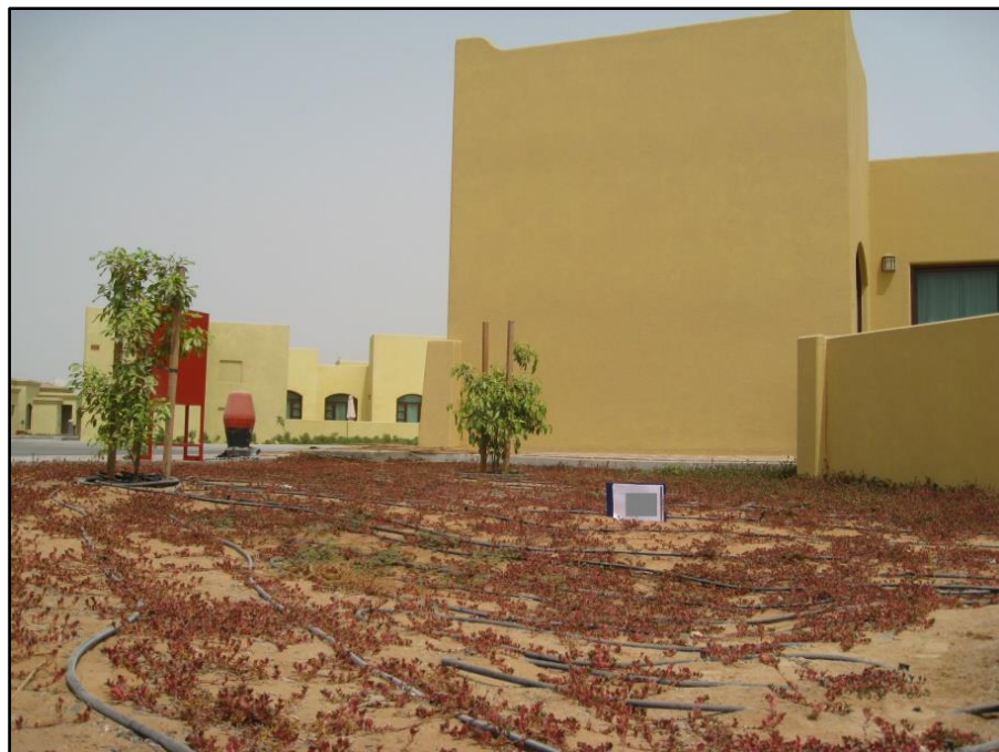
Figure 3.9 Settlement of ground within a landscaped area
