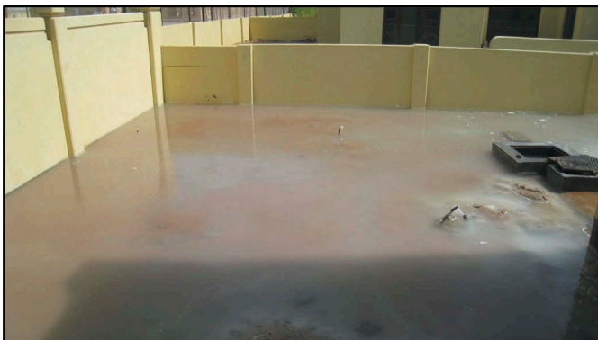
Figure 4. Investigative flooding of landscaped areas.
