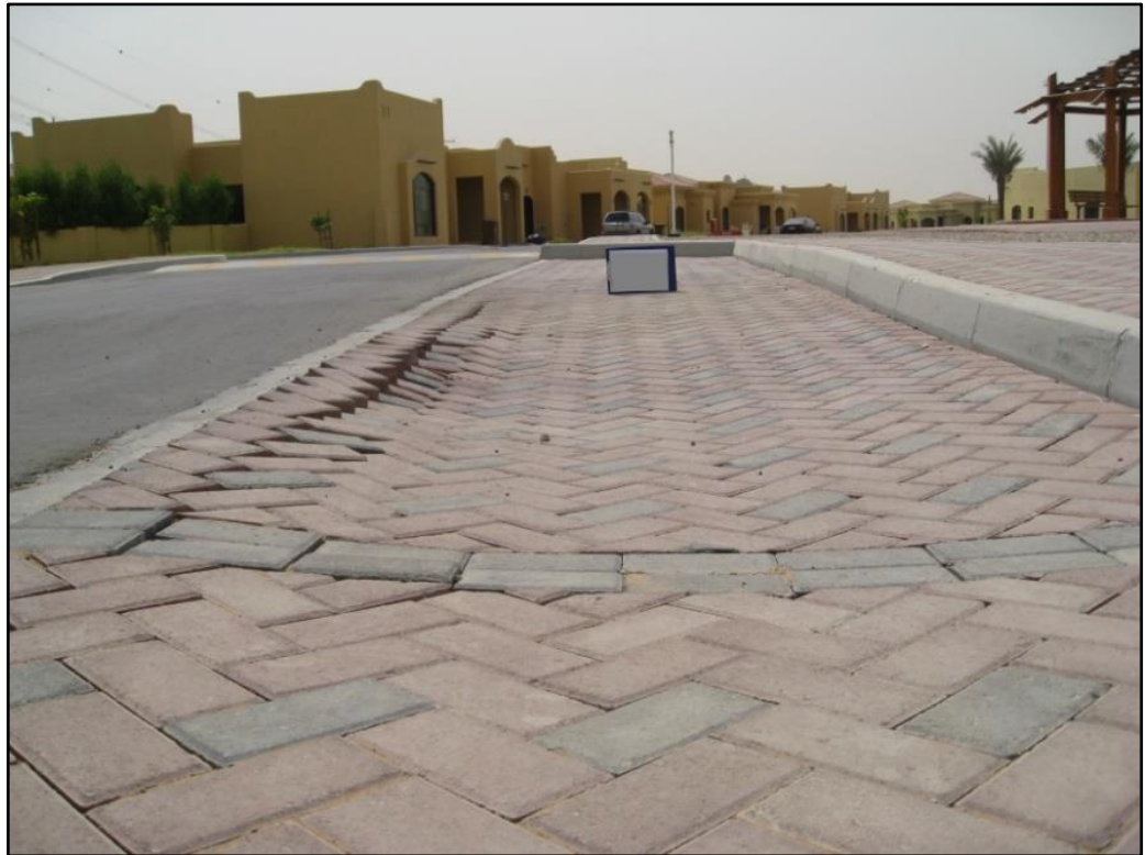
Figure 3.6 Subsidence in paved areas (footpaths)
