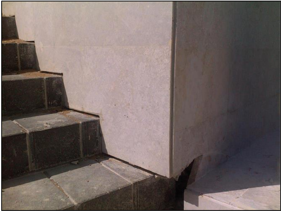
Figure 3.3 Separation of stairs from adjacent wall due to differential settlement
