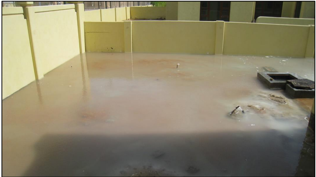
Figure 3.10 Hydro-compaction in progress
