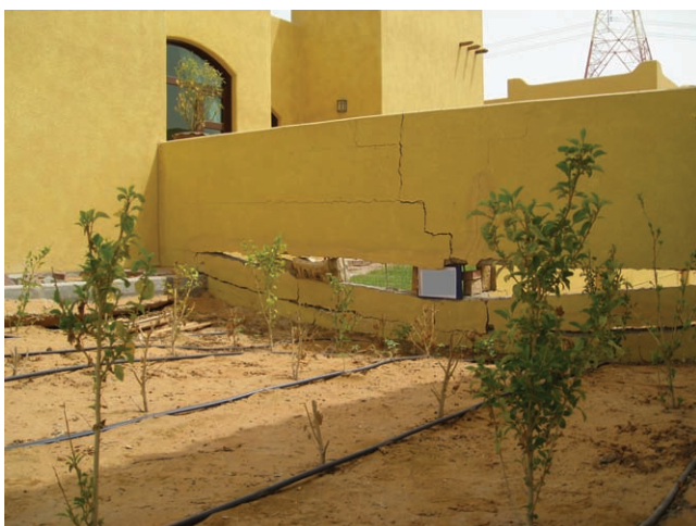
Figure 4. Cracking and settlement of boundary wall
