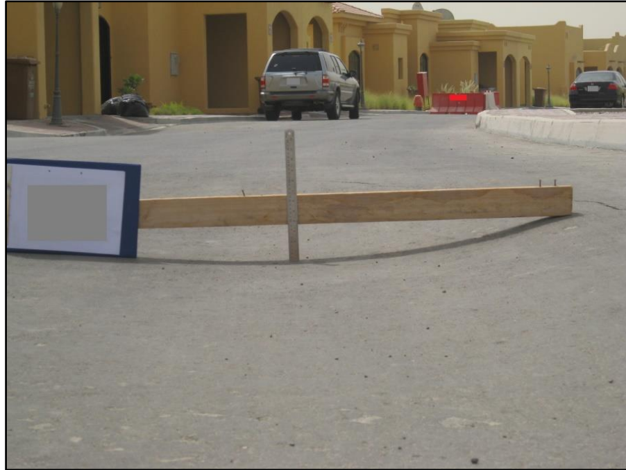
Figure 3.8 Sagging of road
