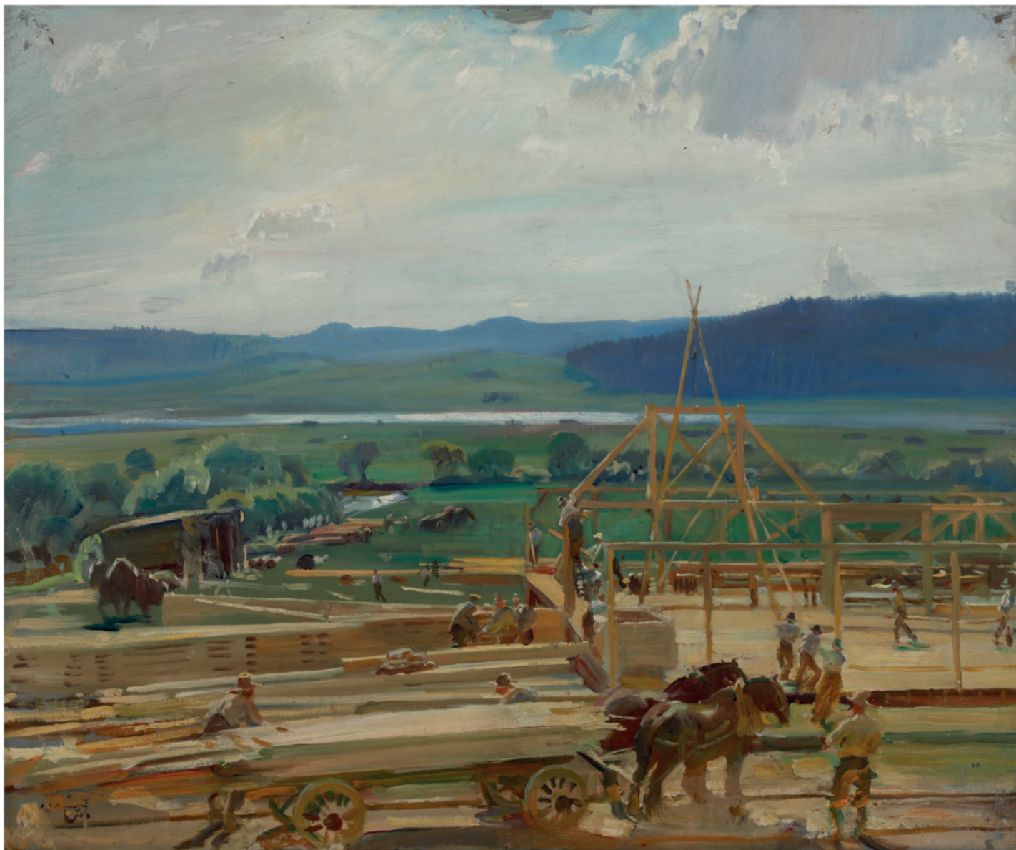
[Plate 34] 36th Company, Canadian Forestry Corps, Building a Mill at Labergement, Jura, 1918, 51 x 61.5 cm (19710261-0472)
