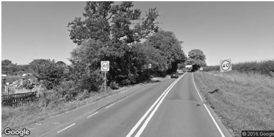
Figure 5.13: Road R3 speed limit reduction and upcoming curve responsible for speed reduction.
