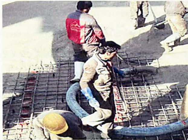
Ready mixed concrete works
