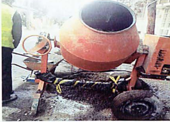
In-situ concrete works
