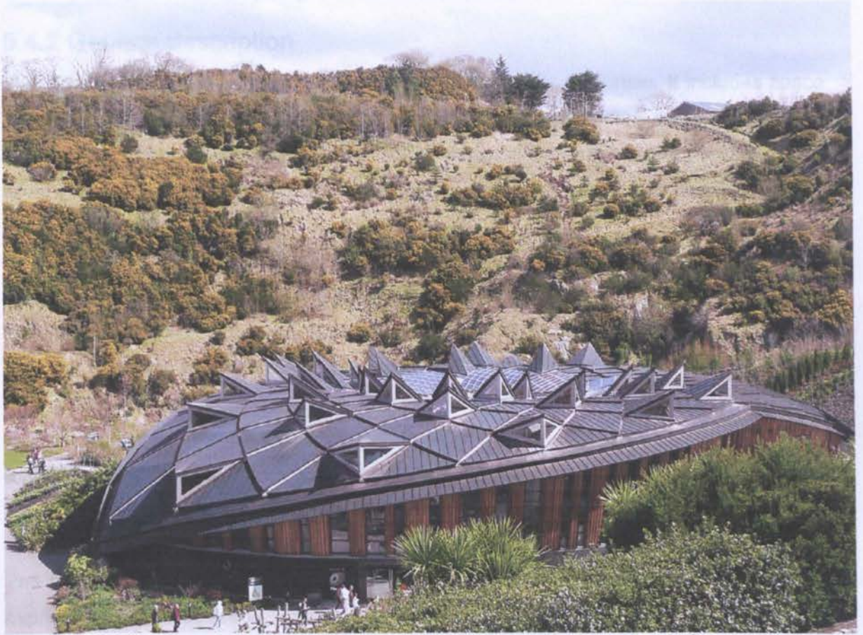
Figure 5.38 The Core building in the context of its surroundings
