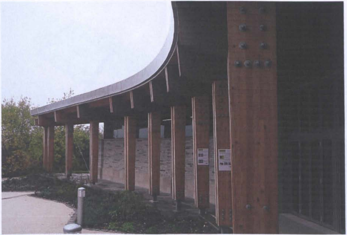
Figure 5.25 Side view of building showing glulam frame and curved design Source: Author
