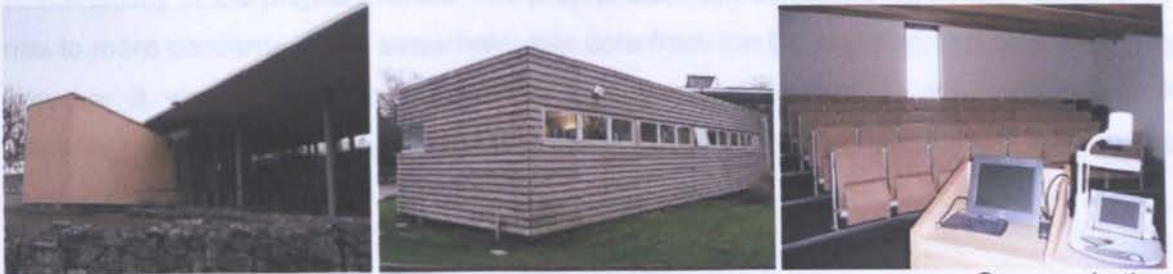
Figure 7.4 Views of the Genesis Project building
