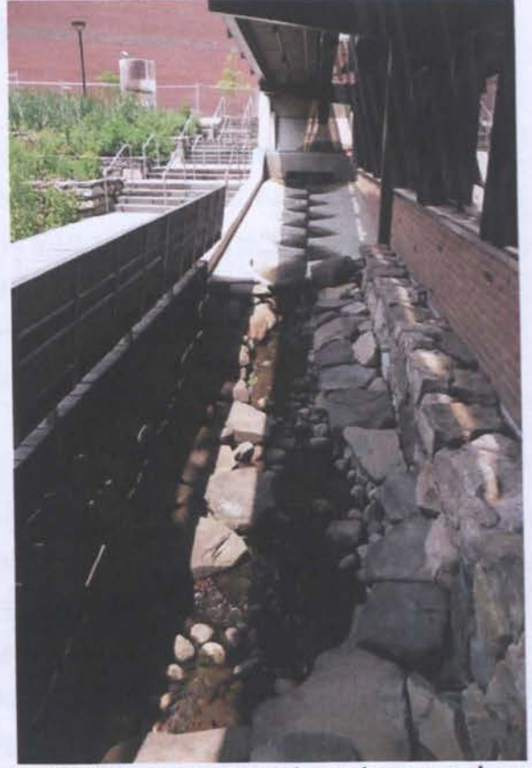
Figure 5.88 Water feature integrated into water management system used as teaching and learning resource. Source: Author
