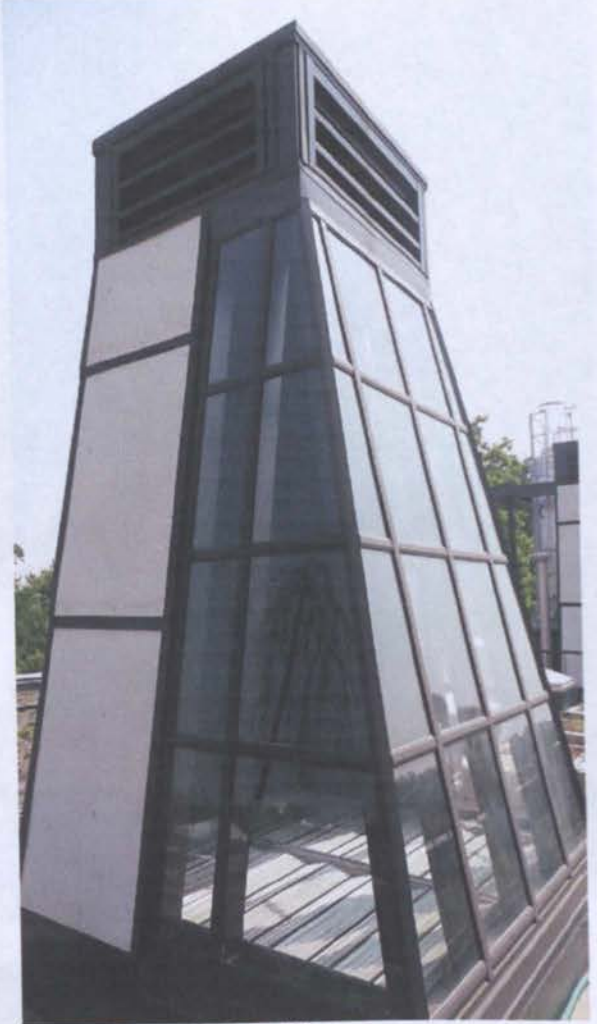
Figure 5.81 Solar chimney. Source: Author
