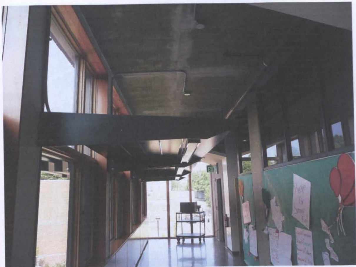
Figure 5.83 Solar reflector in corridor redirecting daylight into classrooms.
