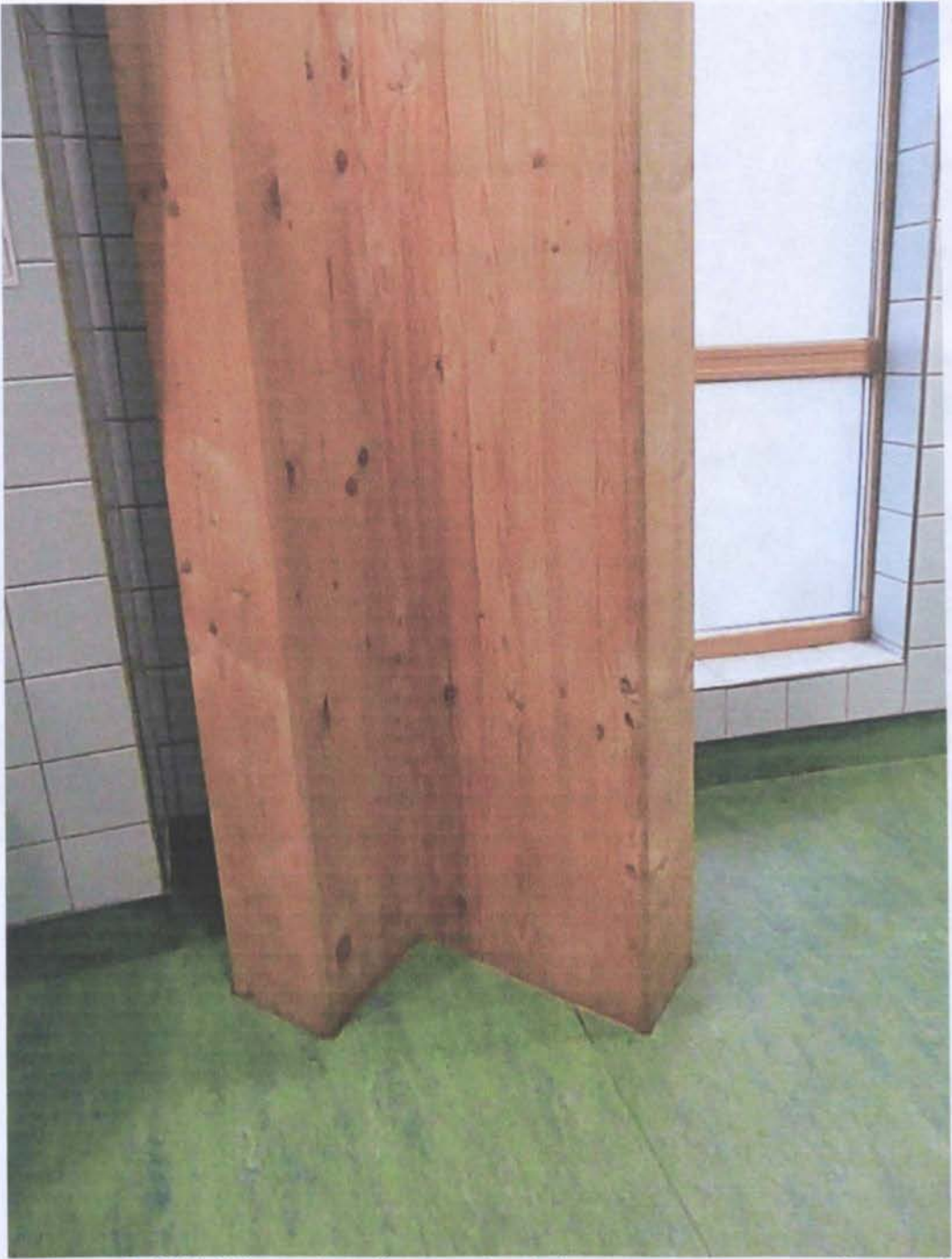
Figure 5.41 Visible and tactile structural element
