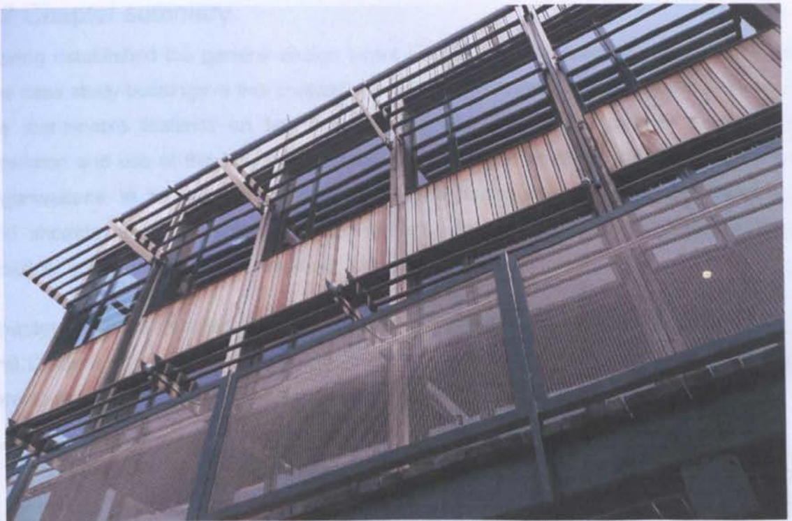
Figure 5.87 View of horizontal solar shading device. Source: Author
