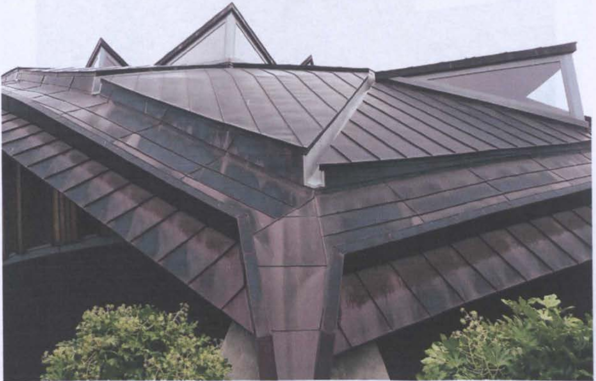
Figure 5.39 The sustainably sourced copper roof
