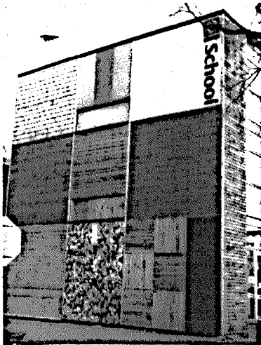
Figure 3.15 Rear view of building Source: Author
