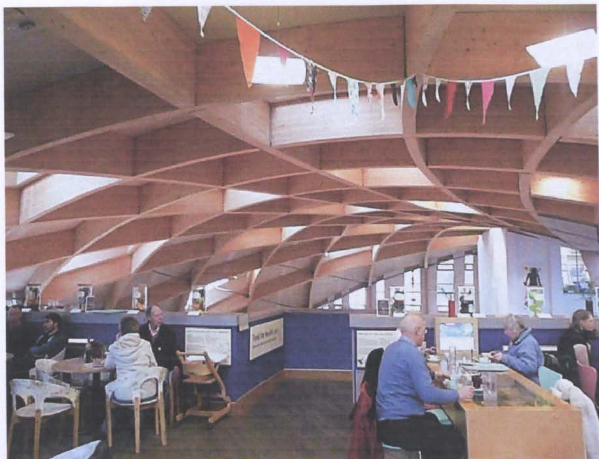
Figure 5.42 Visitor cafeteria under visible roof system
