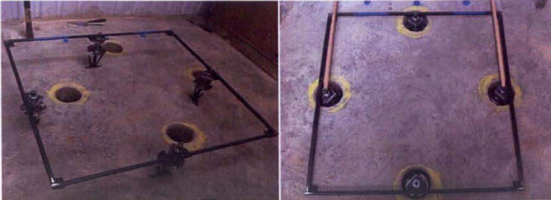
**Figure 3-13 Steel frame for placing inserts in the holes**
