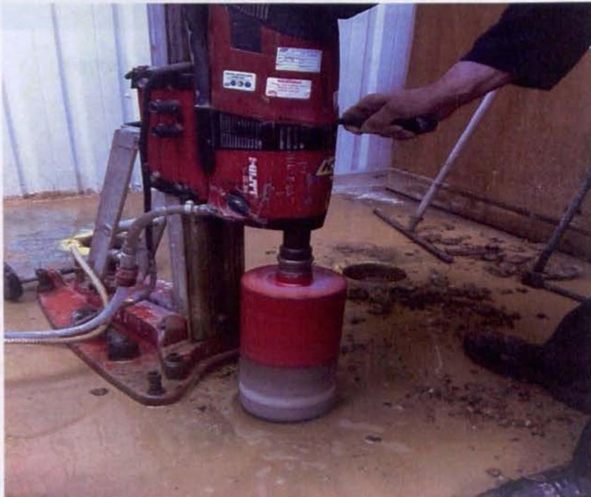
Figure 3-12 Drilling holes for the slab testing rig
