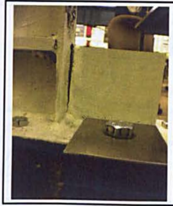
Figure 6.27: Weld fracture and formation of plastic hinges at end of the column
