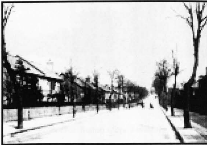
Figure 6.15 Cavendish Road, 1890s
