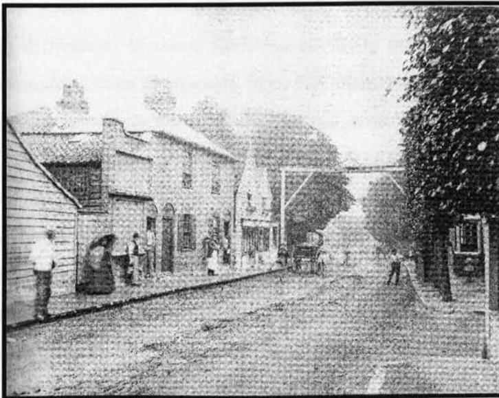
Figure 5.1 The poor state of the High Street looking downhill and northwards towards The Greyhound Inn in the 1860s
