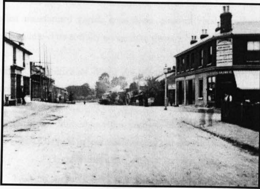
Figure 4.14 Filling the housing gaps - in Lind Road, Newtown
