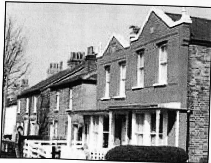
Figure 6.20 Victoria Cottages and Jubilee Villas, Lind Road
