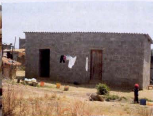
A Completed House.
