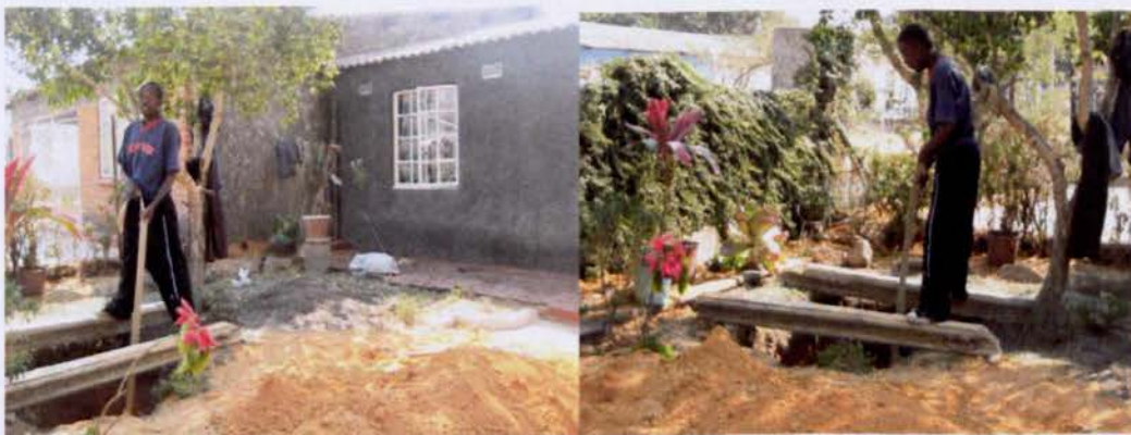
Digging for Water in the Front Garden.
