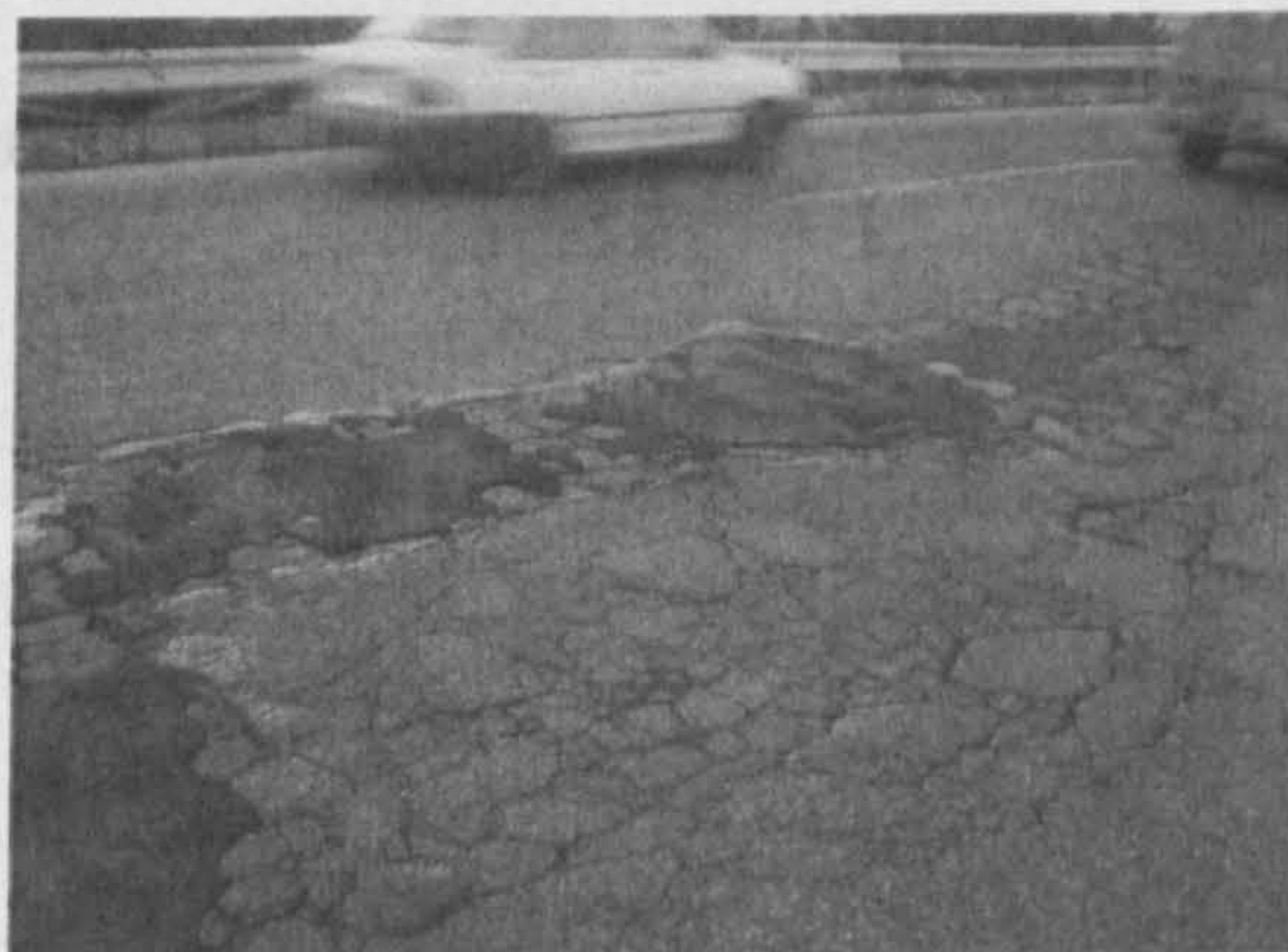
Figure 4.29 Asphalt distresses
