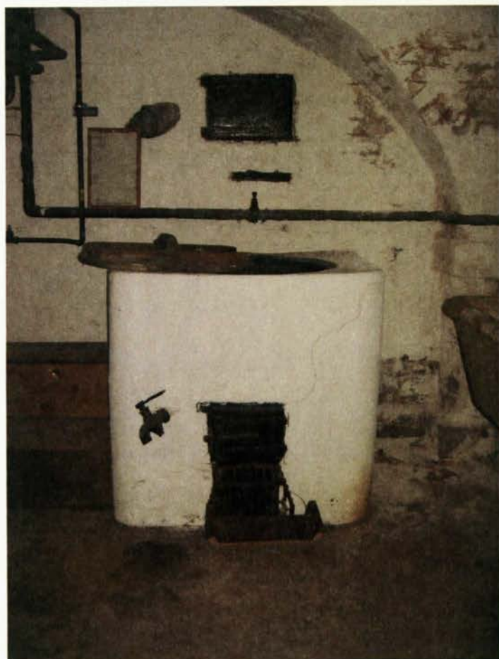
Figure 105. Inbuilt copper for heating water, located in the basement of the German kitchen, Hampton Court Palace, author photograph, 2011.
