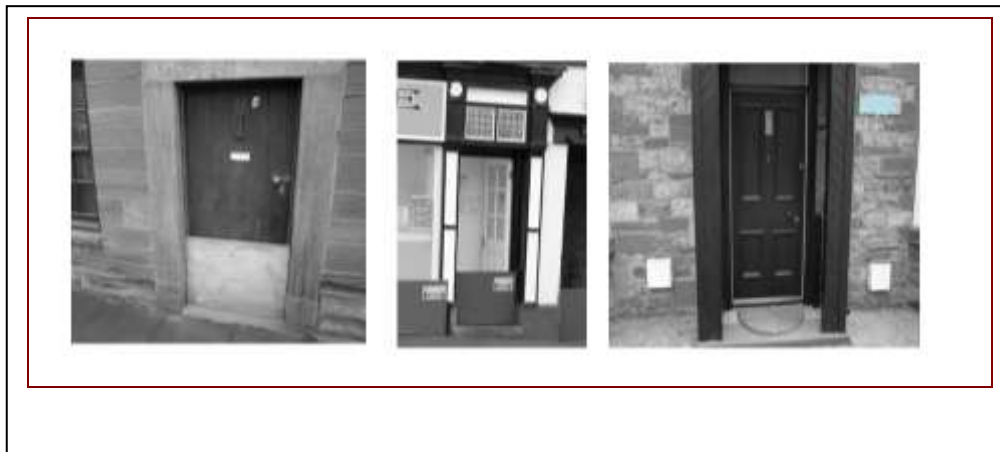
64 Figure 1 Examples of protection measures: a home-made door-board, a commercial door- 65 board and commercial airbrick covers
