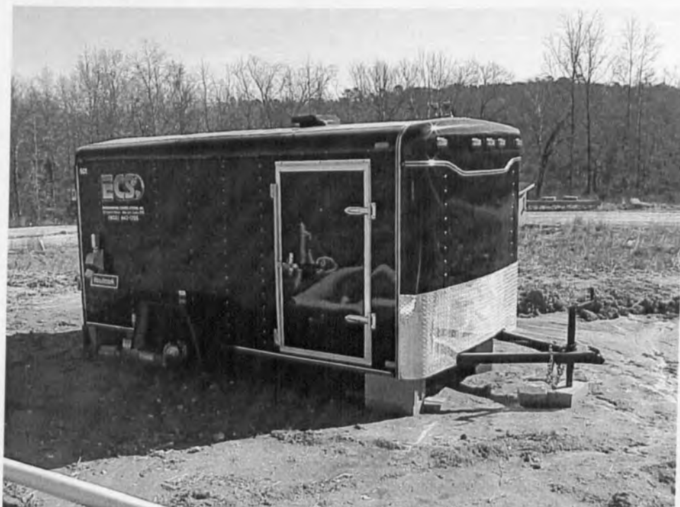
Figure 6. Automated Control Centre for Landfill Site Number 1 (source: author)
