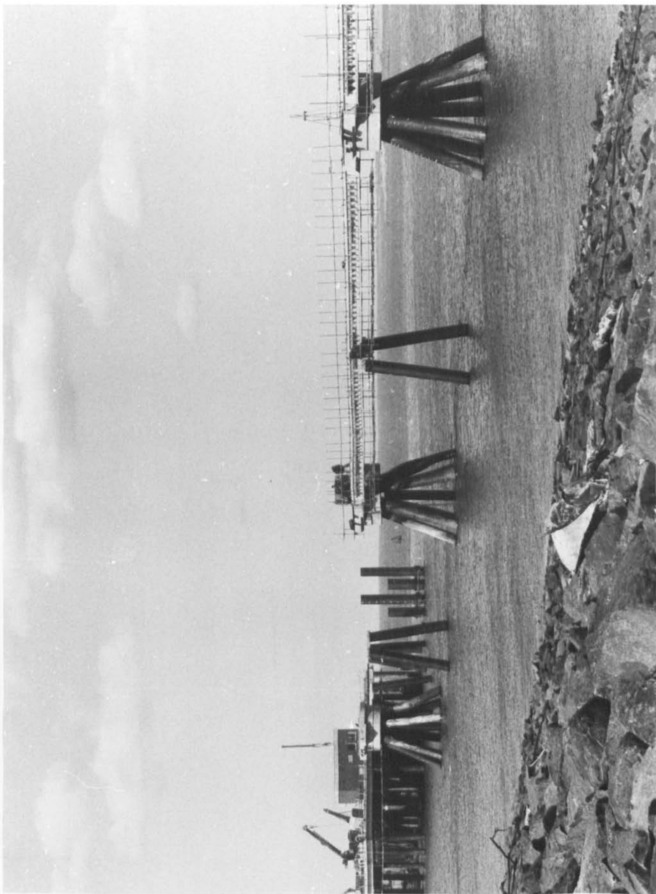
Figure 8 - Jetty Construction - CHS Piles
