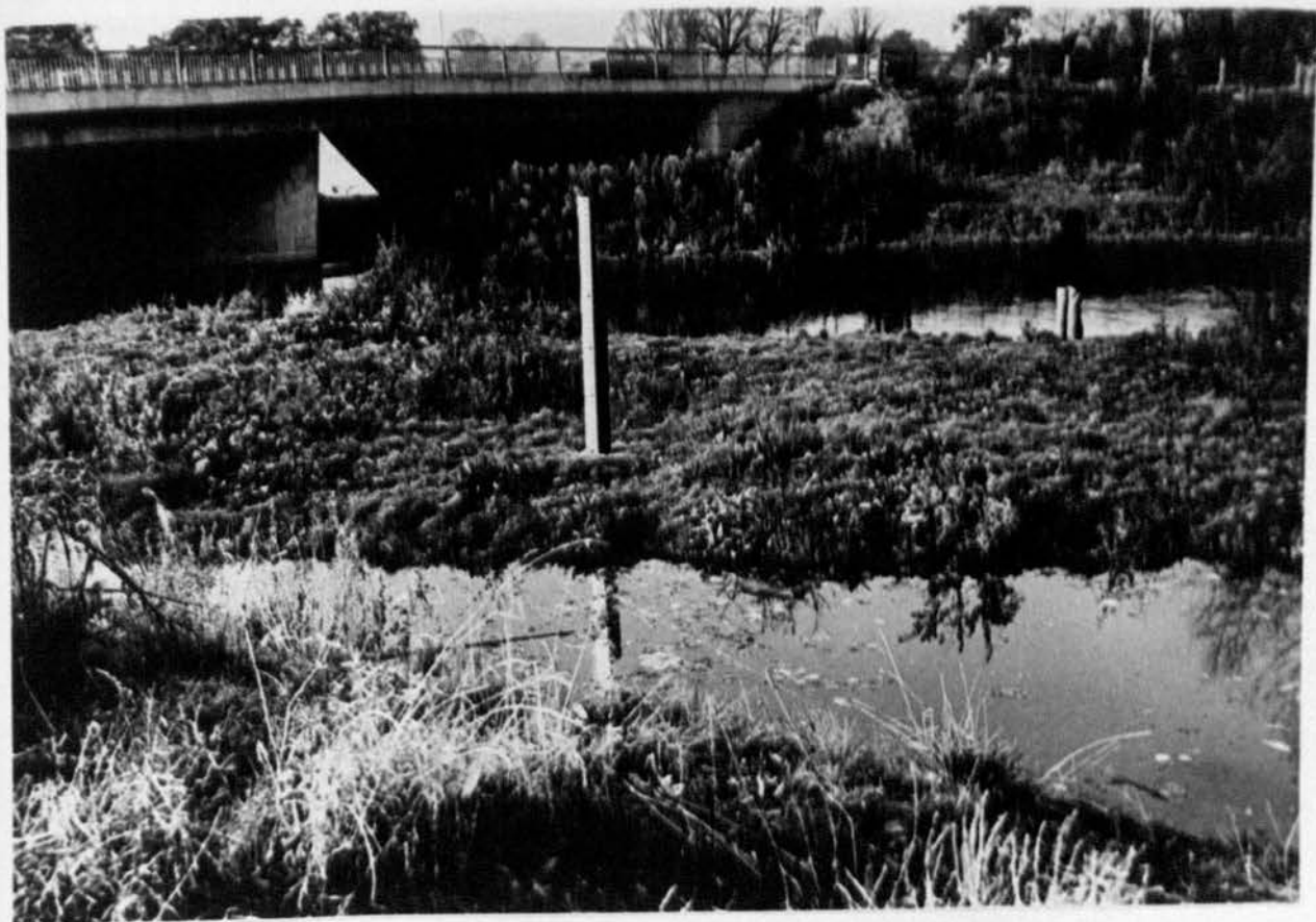
Plate 33. New Downside Bridge and Gauge Board - Low Flow.
