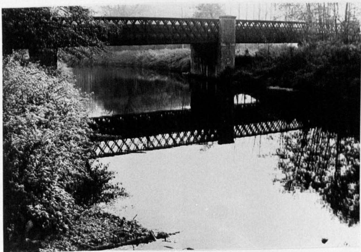
Plate 27. Site of Level Recorder at Downside Mill and Downside Rail Bridge.
