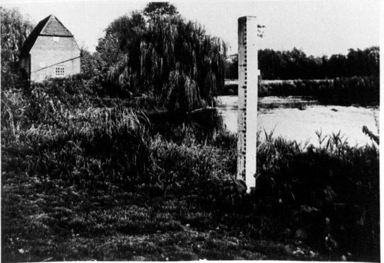
Plate 30. Channel Downstream of Cobham Mill.
