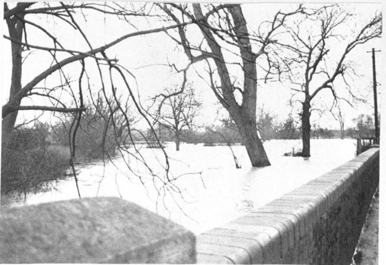
Plate 8. Flooding Upstream of Flanchford Bridge - Event 32.
