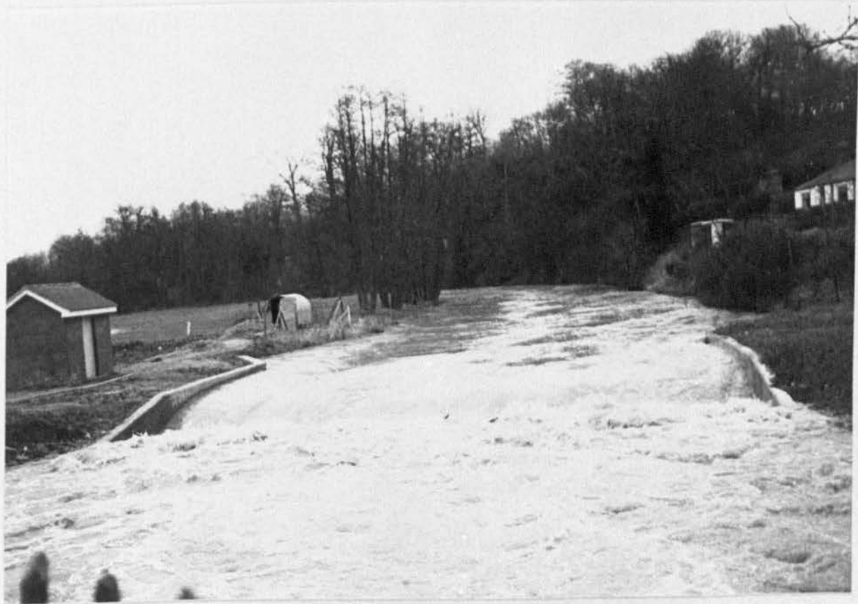
Plate 19. New Crump Weir at Castle Mill - Event 32.
