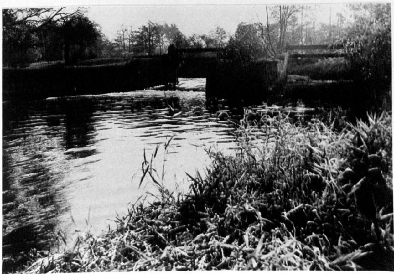
Plate 28. Downside Mill Weir.
