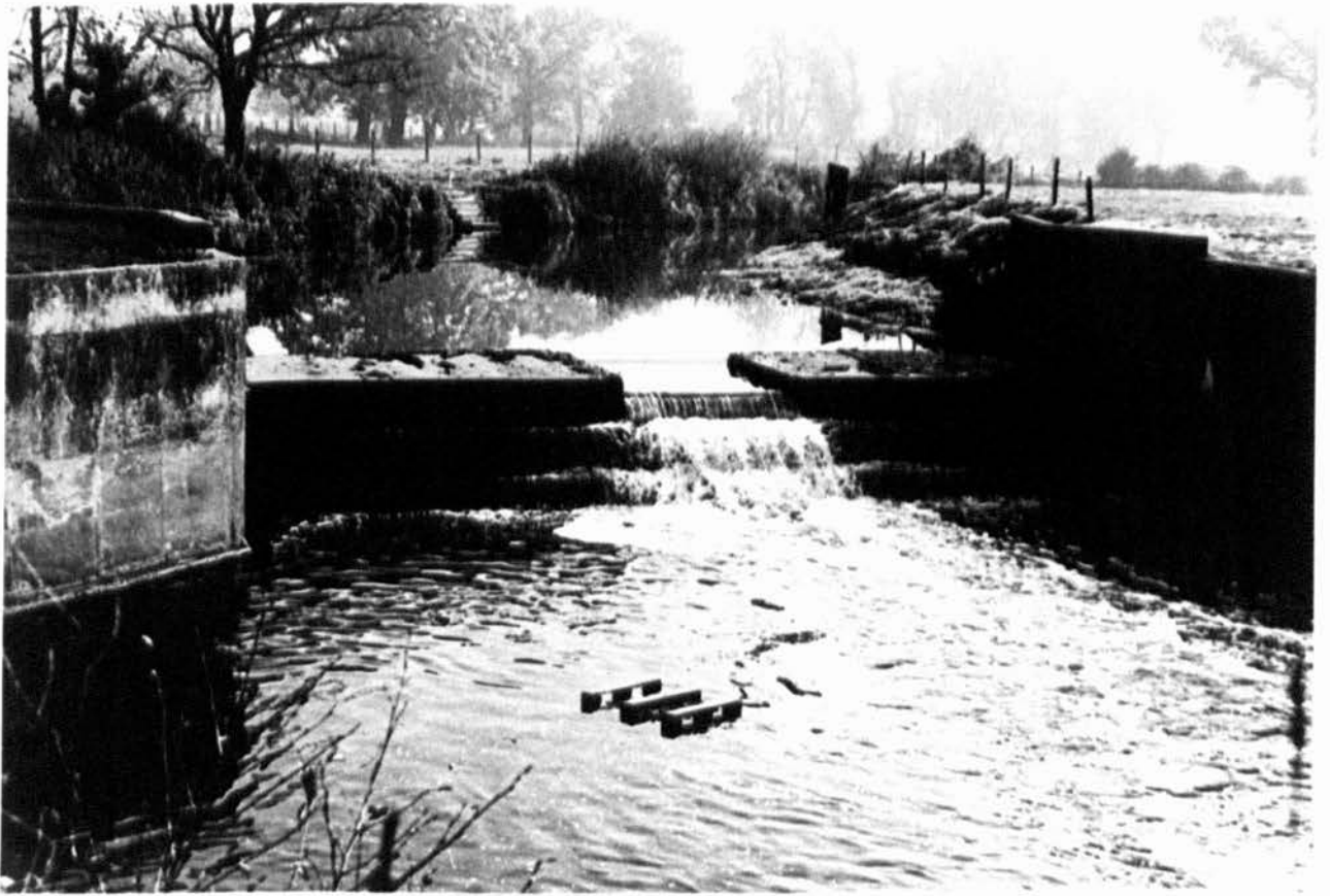
Plate 1. Horley Gauge Weir and Head Water Level Recorder.
