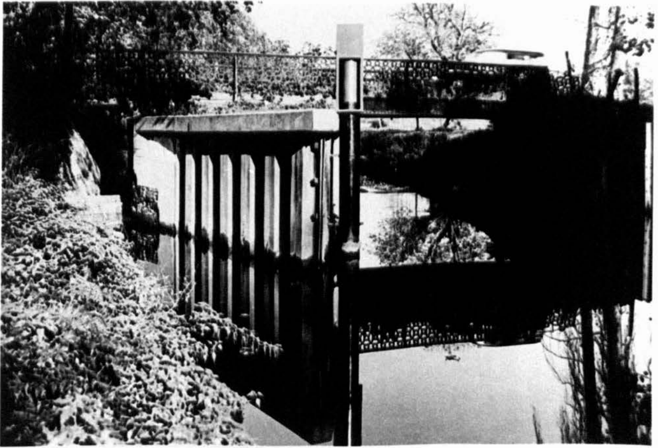
Plate 3. Kinnersley Manor Weir and Head Water Level Recorder.
