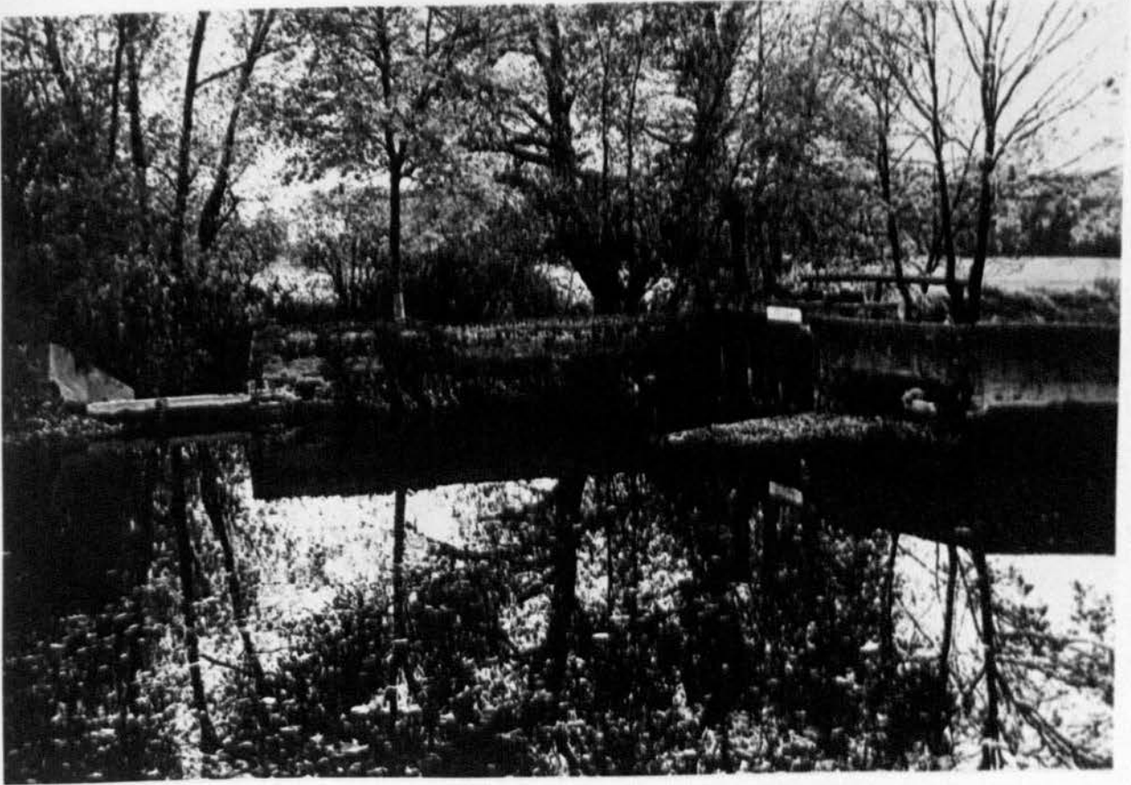
Plate 29. Cobham Mill Sluices.
