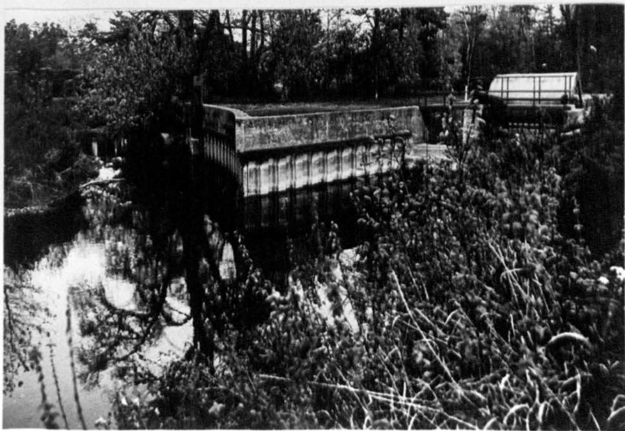
Plate 46. Wilderness Sluice Gates.
