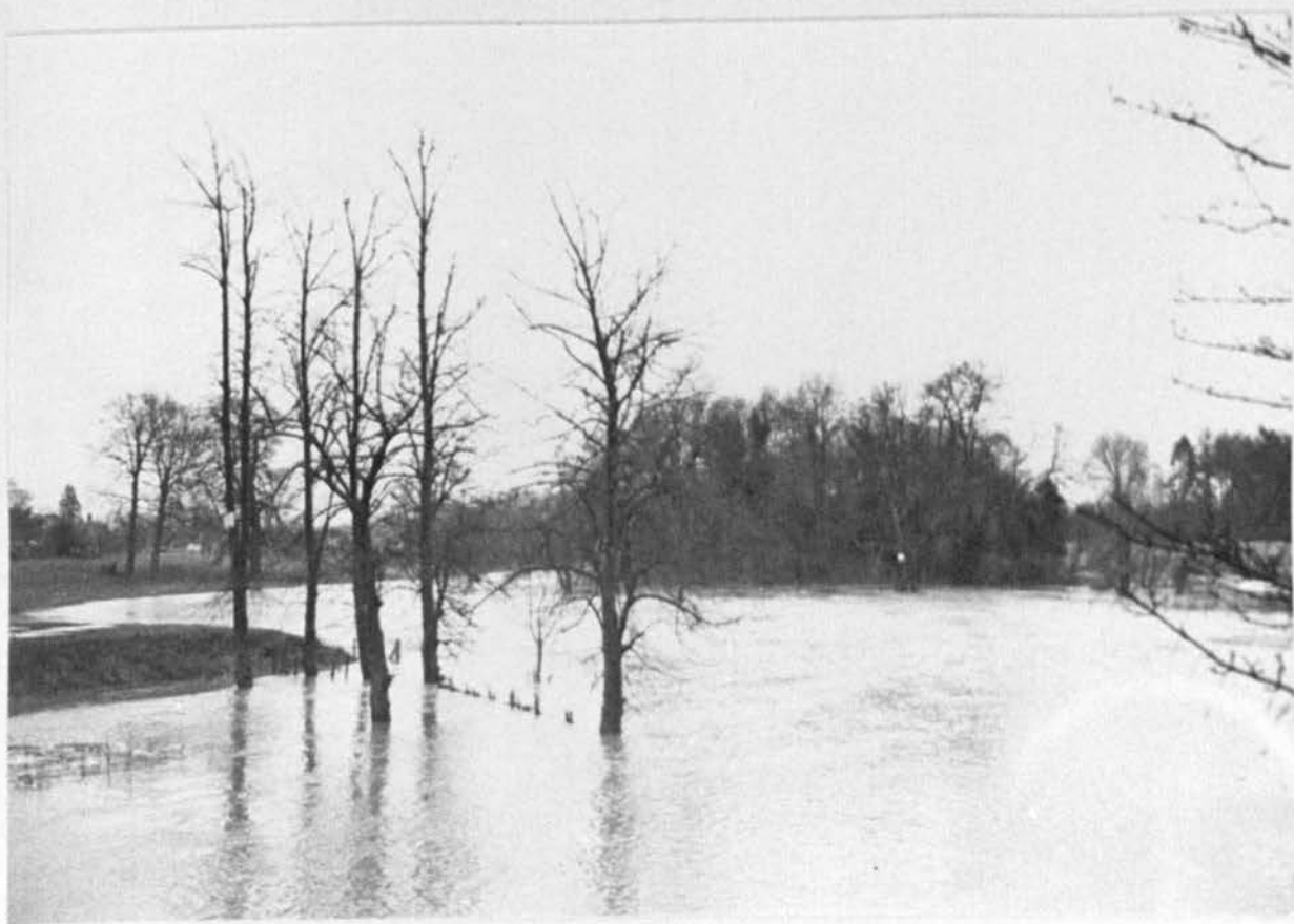
Plate 38. Painshill Weir Drowned Out and Flooding Upstream of Cobham Bridge - Event 32.
