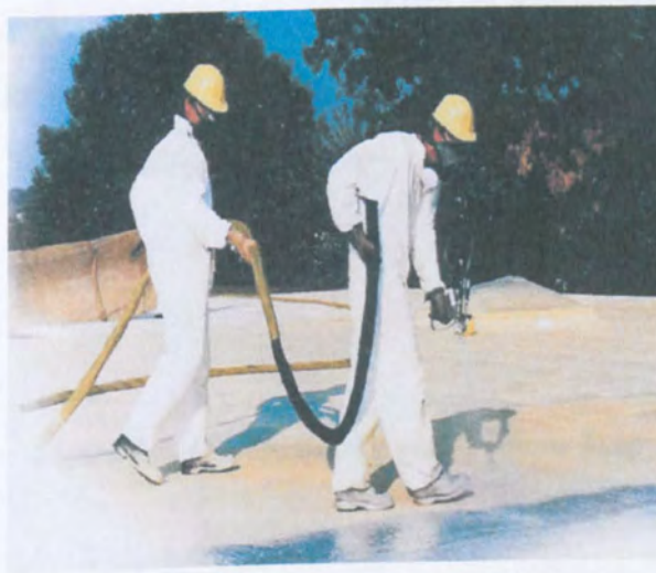
Fig 3.7: Polyurethane being sprayed on roofs [45]
