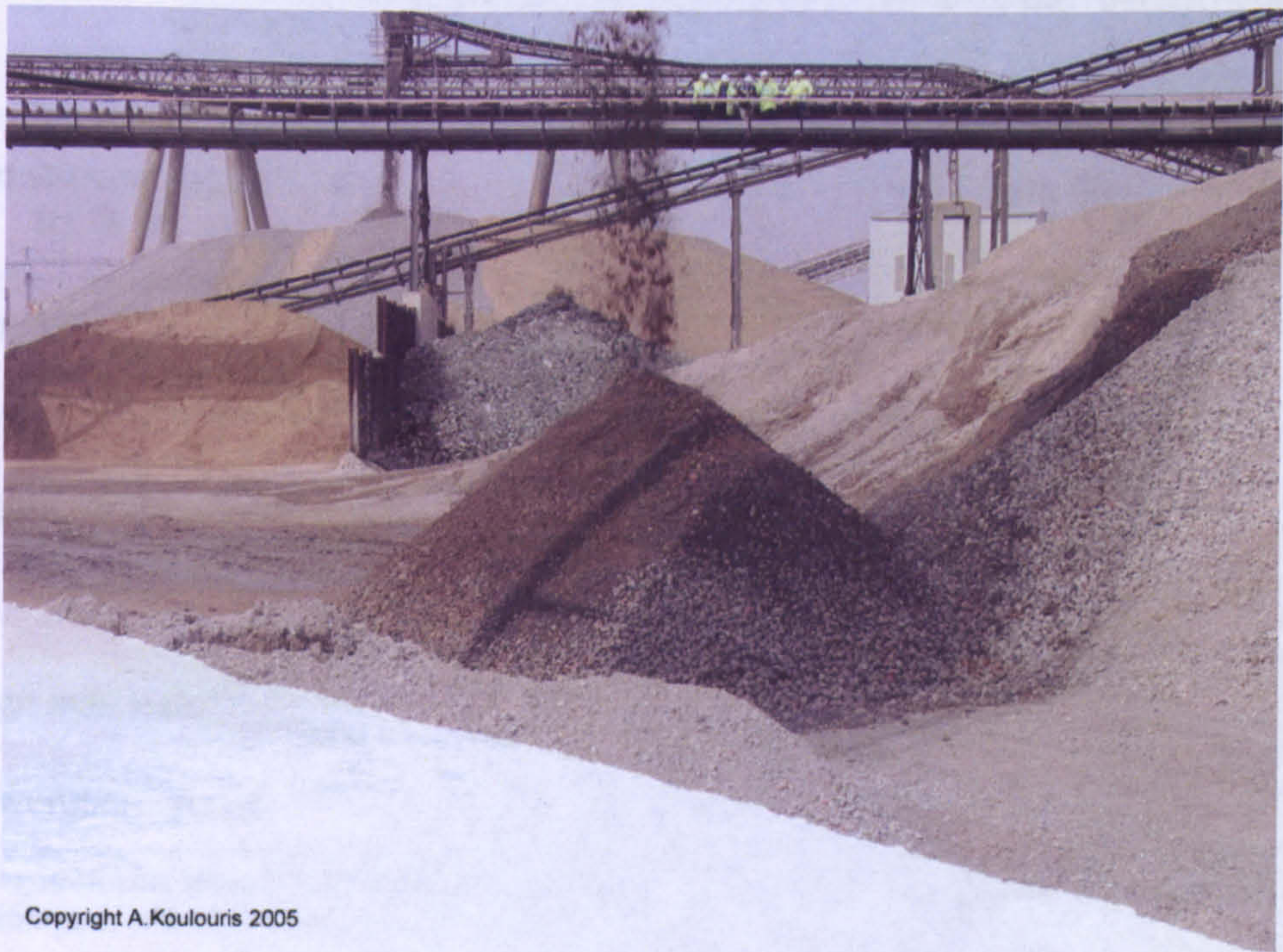
Figure 4.6 Stockpile of the clean and graded coarse RCA produced at the recycling plant.
