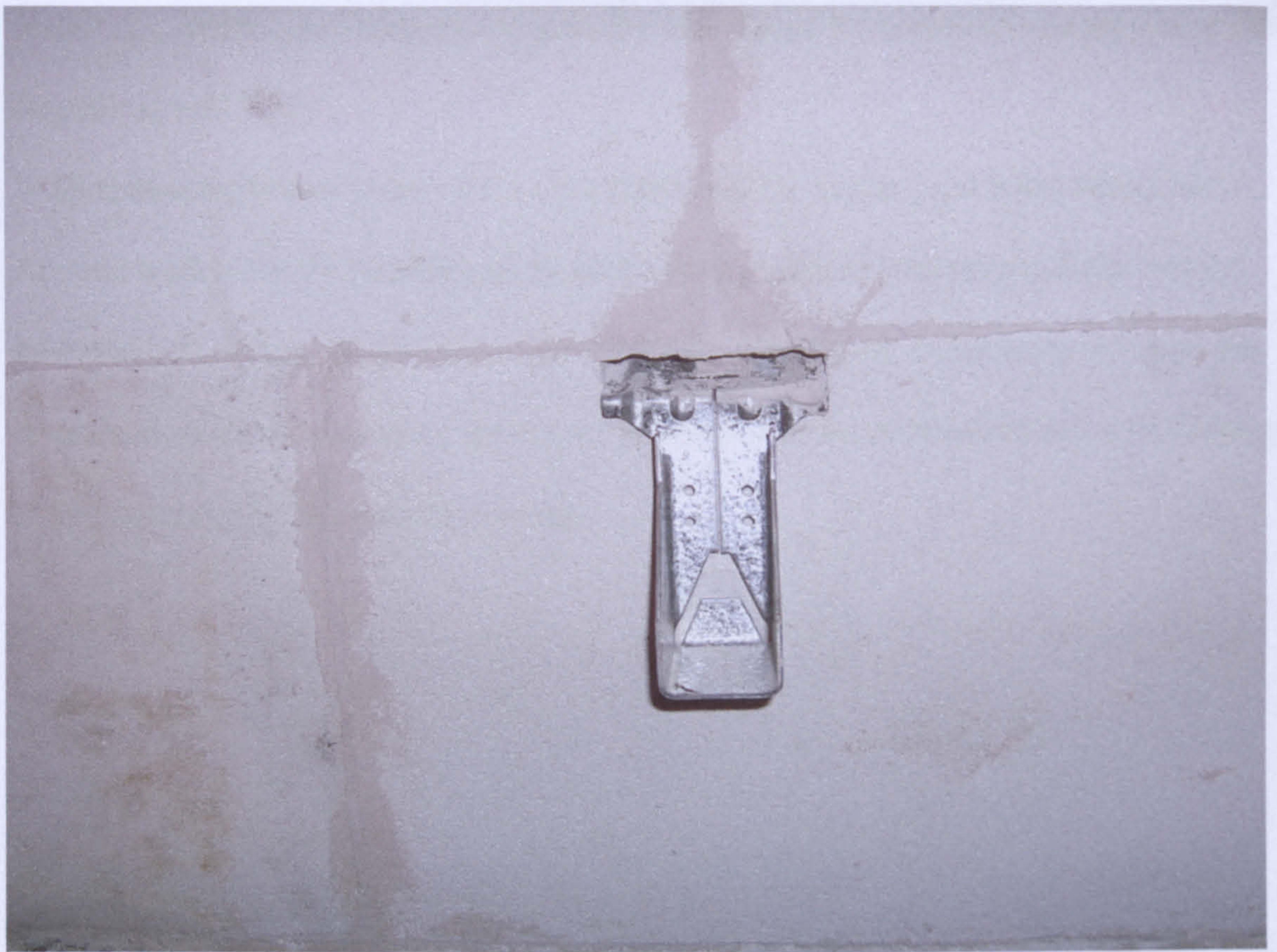
Figure 46: Failure of joist hanger using metal joist
