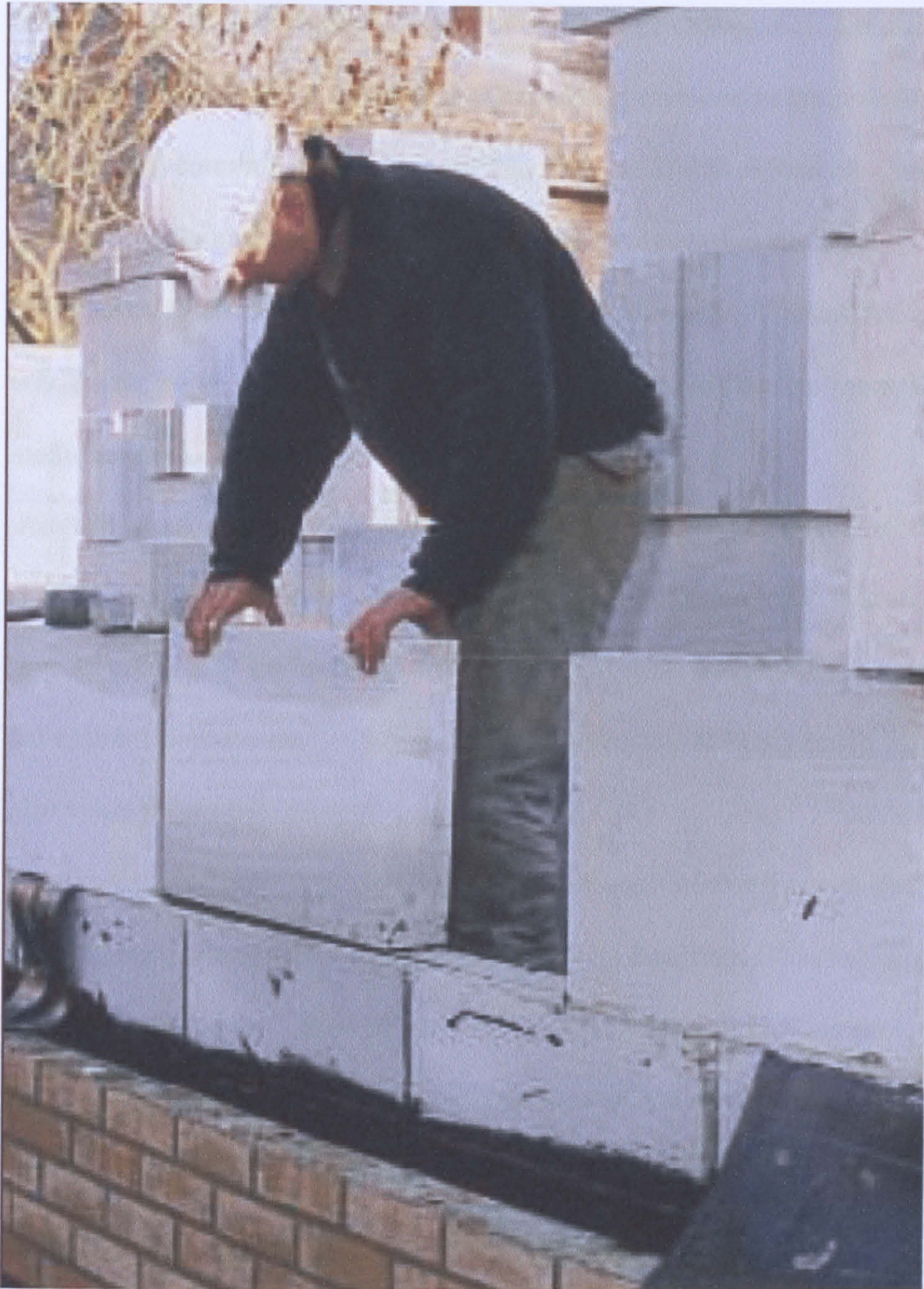
Figure 1: Laying Aircrete blocks in thin layer mortar
