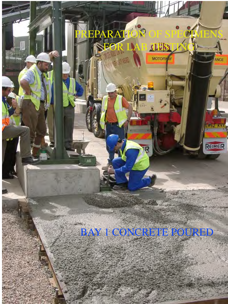
Figure 9.3: Specimen preparation during concrete pouring.
