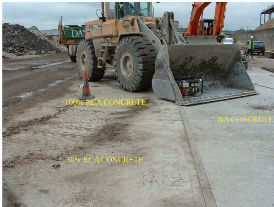
Figure 9.6: Location selected for RCA concrete pavements.
