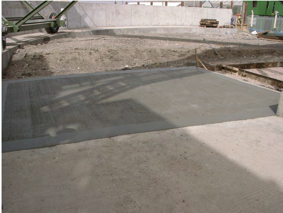
Figure 9.5: Completed pavement using 100% RCA concrete.
