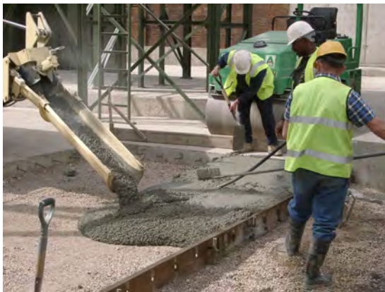
(a) Placing concrete.
