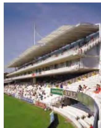
Photograph courtesy of the Concrete Society
