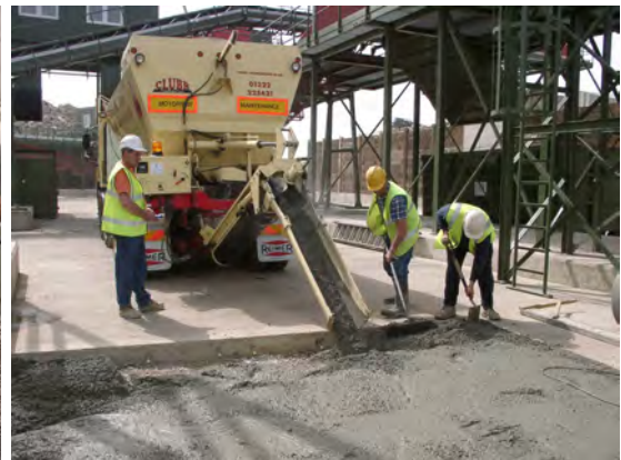
(b) Placing concrete.
