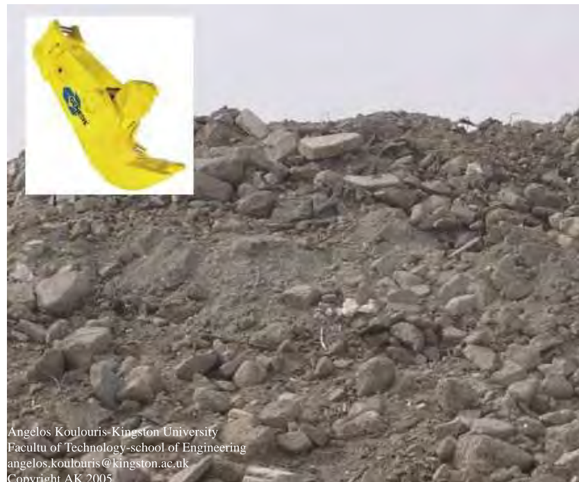
Figure 5.1: C&D debris reduced to a maximum of 0.4 m using hydraulic shears.
