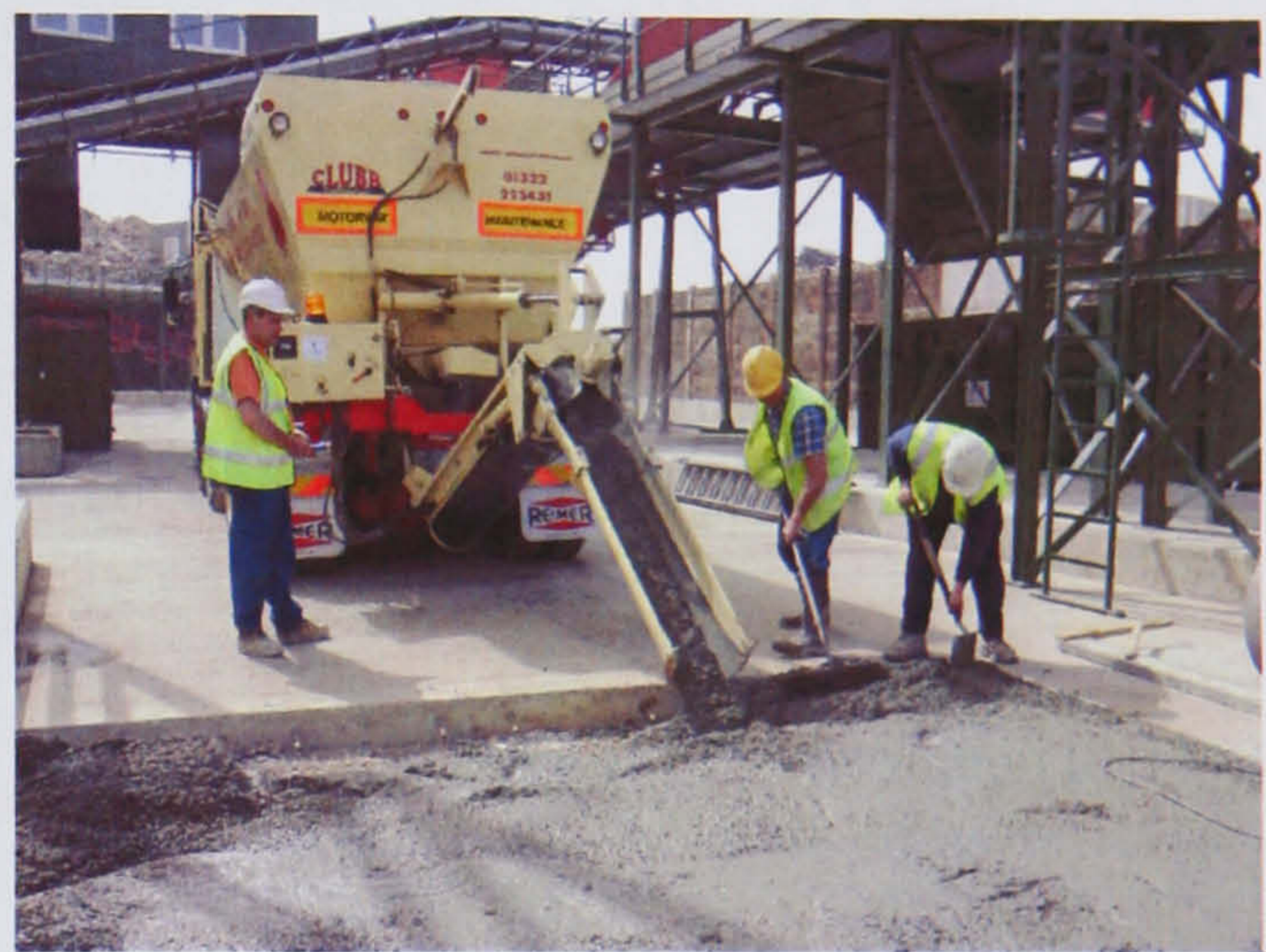
(b) Placing concrete.
