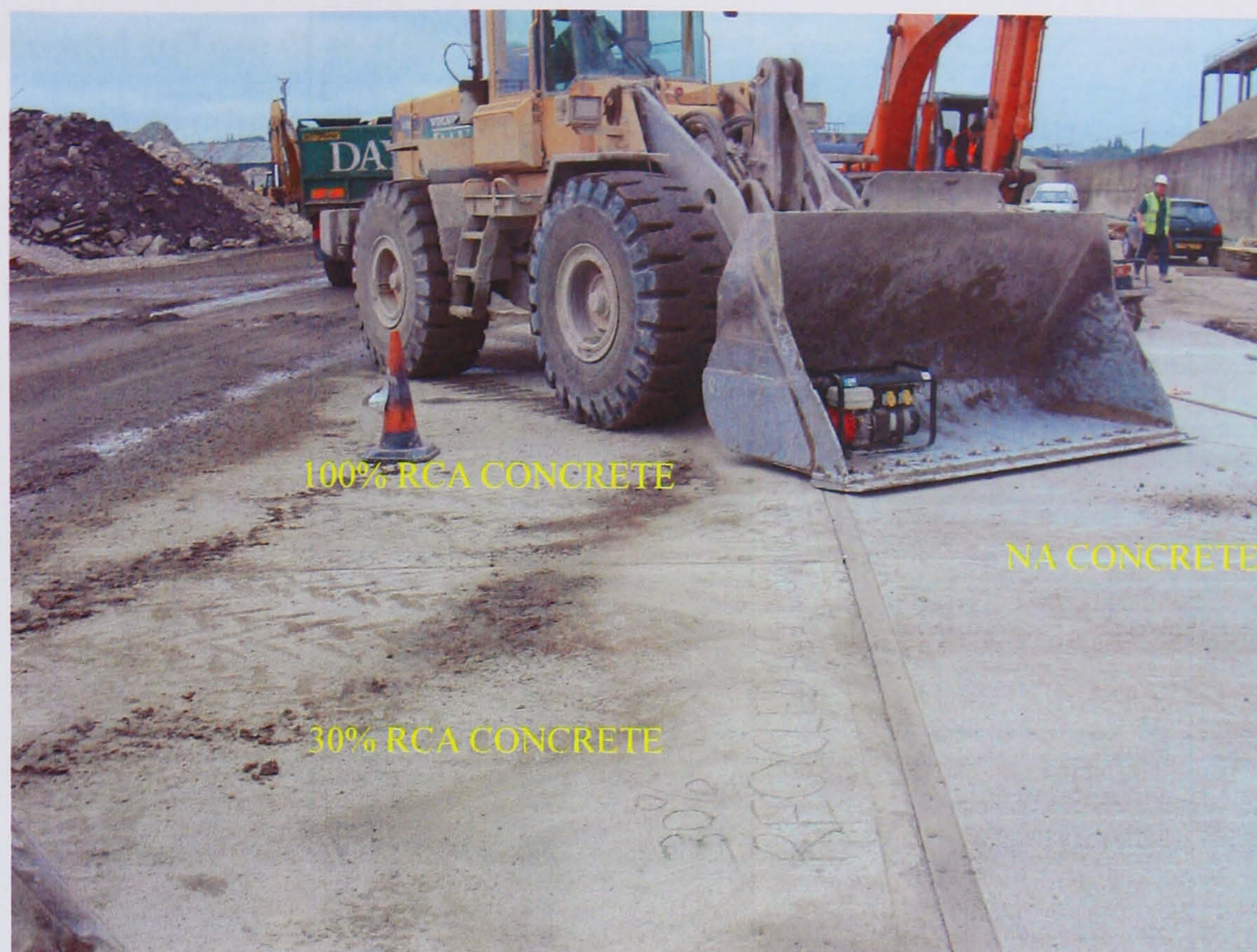
Figure 9.6: Location selected for RCA concrete pavements.
