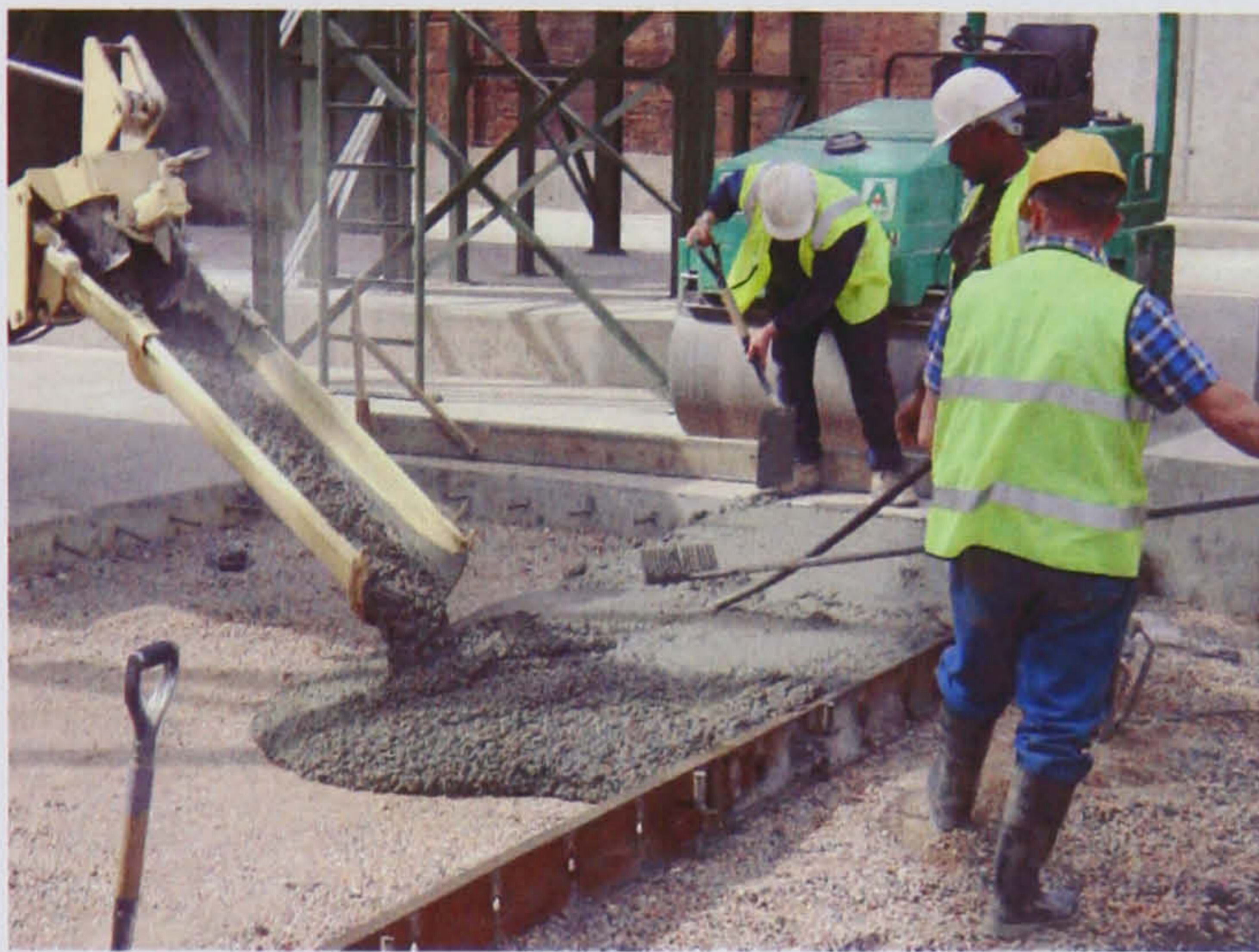
(a) Placing concrete.
