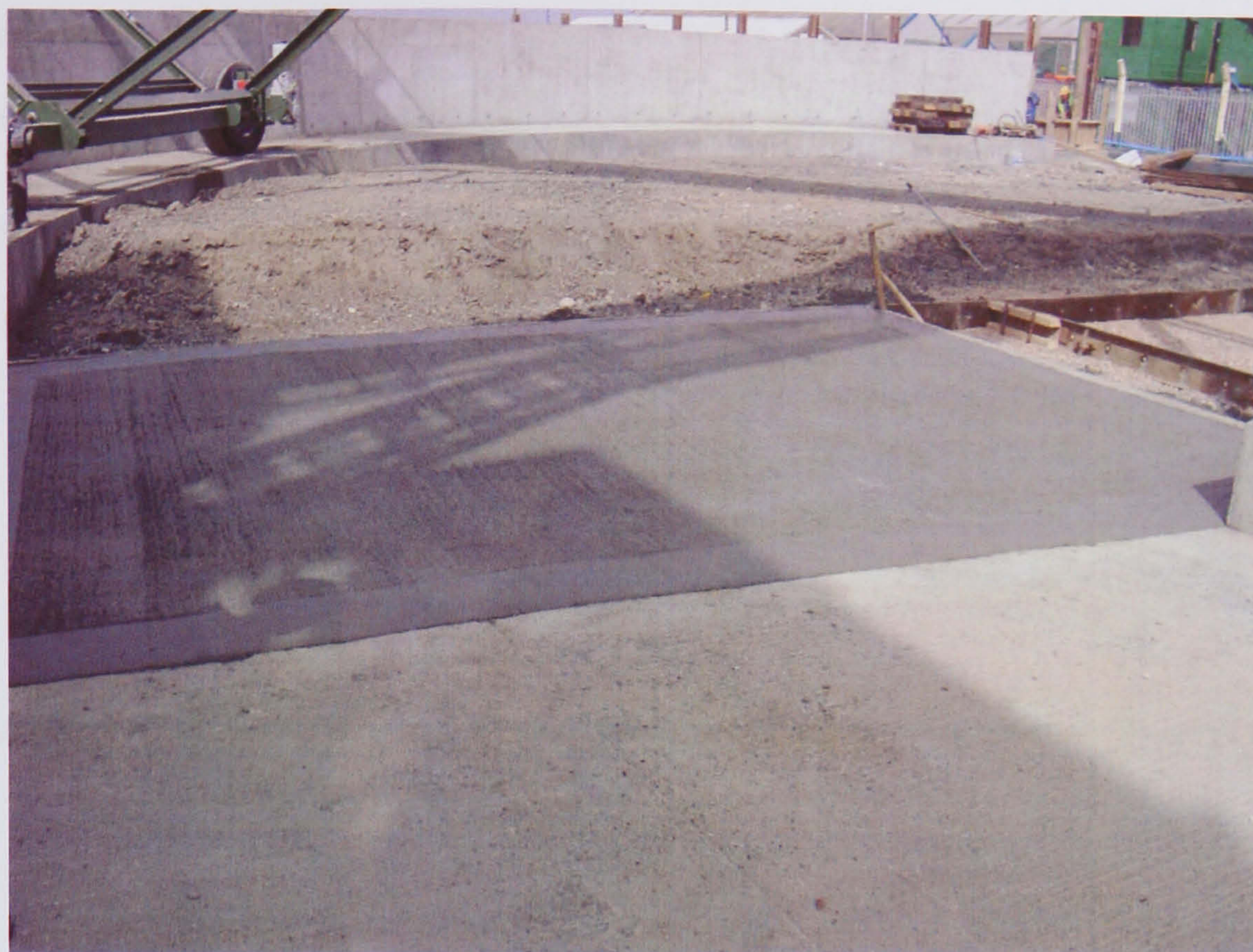
Figure 9.5: Completed pavement using 100% RCA concrete.
