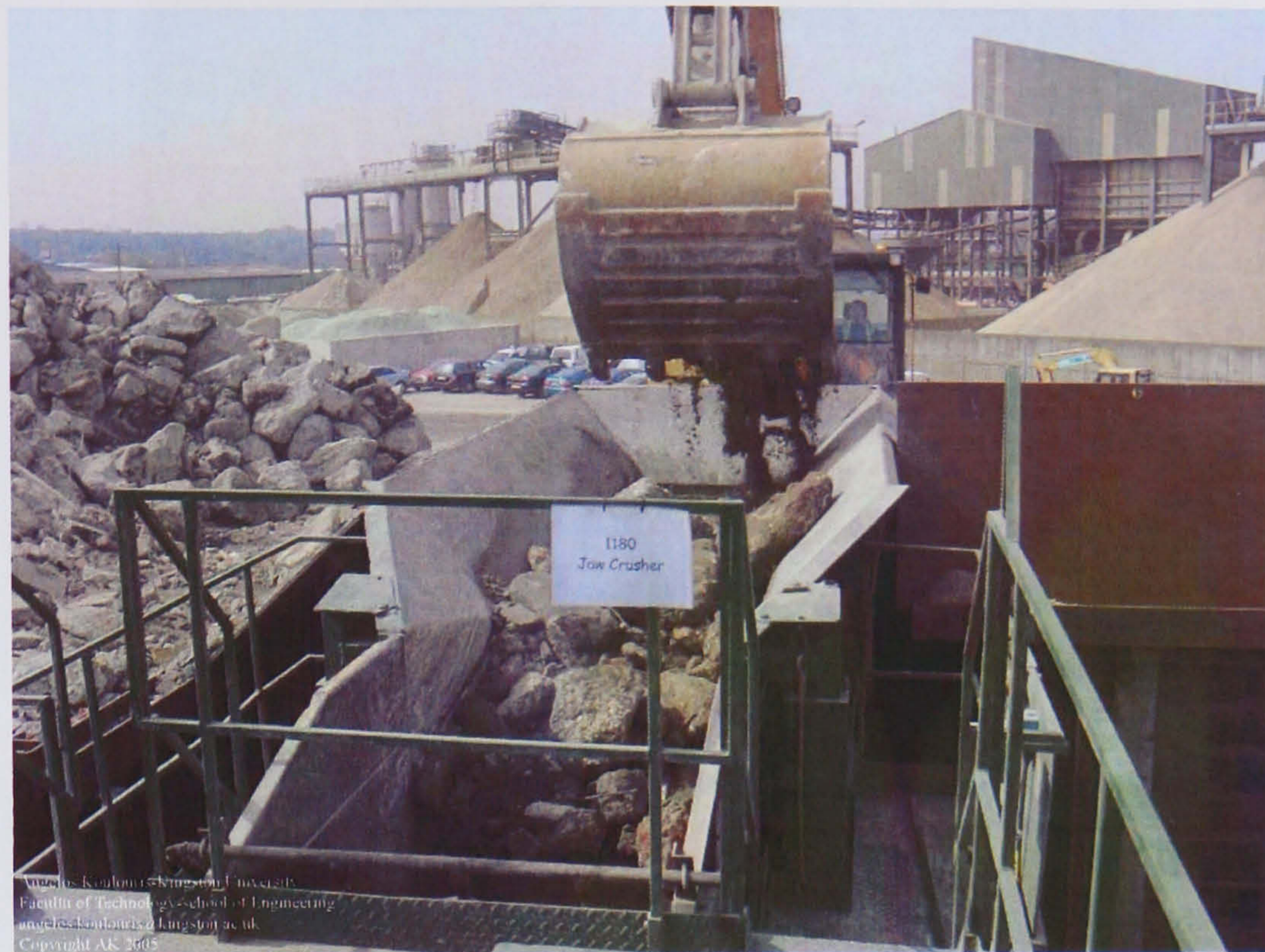
Figure 5.2: Primary jaw crusher loaded with concrete following the process using shears.
