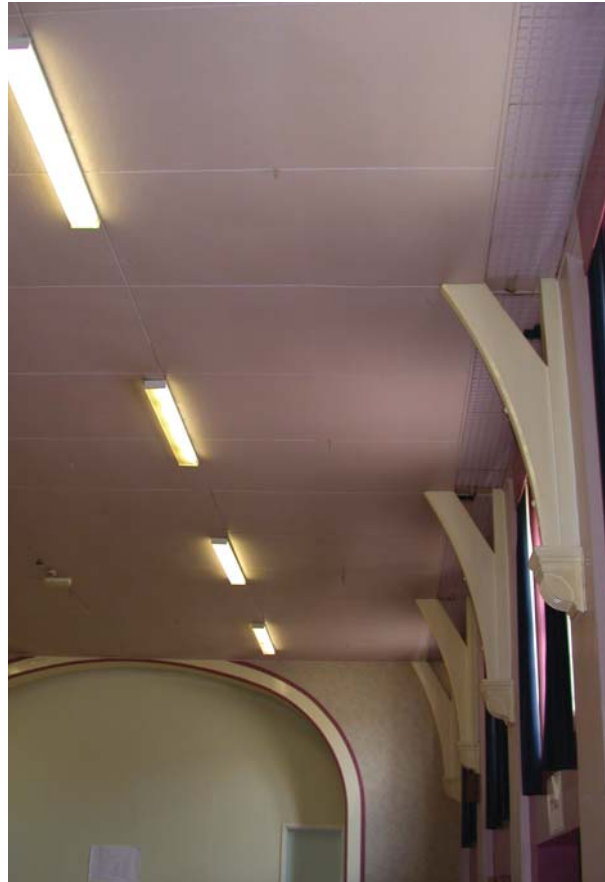
The ceiling before and after structure was exposed
