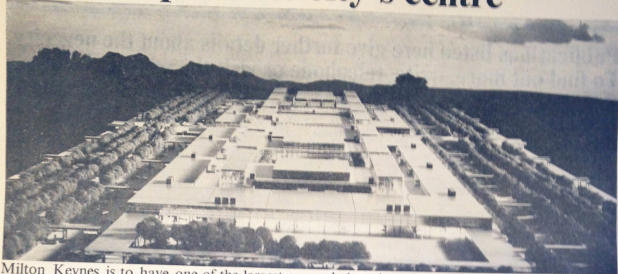
Milton Keynes is to have one of the largest covered shopping areas in Europe and this is it; The Shopping Building. Above is a model showing how the completed building will look. Below is a recent helicopter shot. The building will be nearly half a mile long and will have over 150 shops and catering and entertainment facilities.
