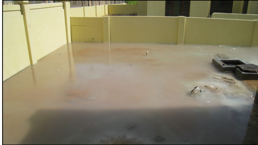
4 Investigative flooding of landscaped areas
