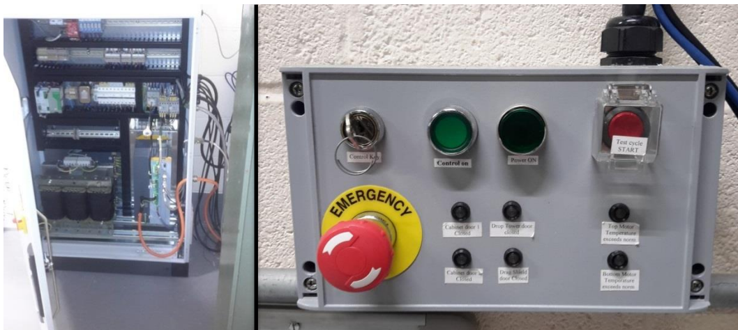
Figure 3.1.4: Electronics cabinet and Control unit
