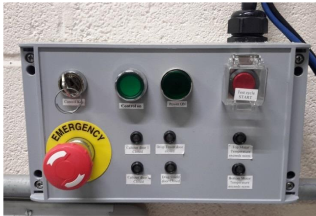
Figure 3.3.19: Drop Tower control panel
