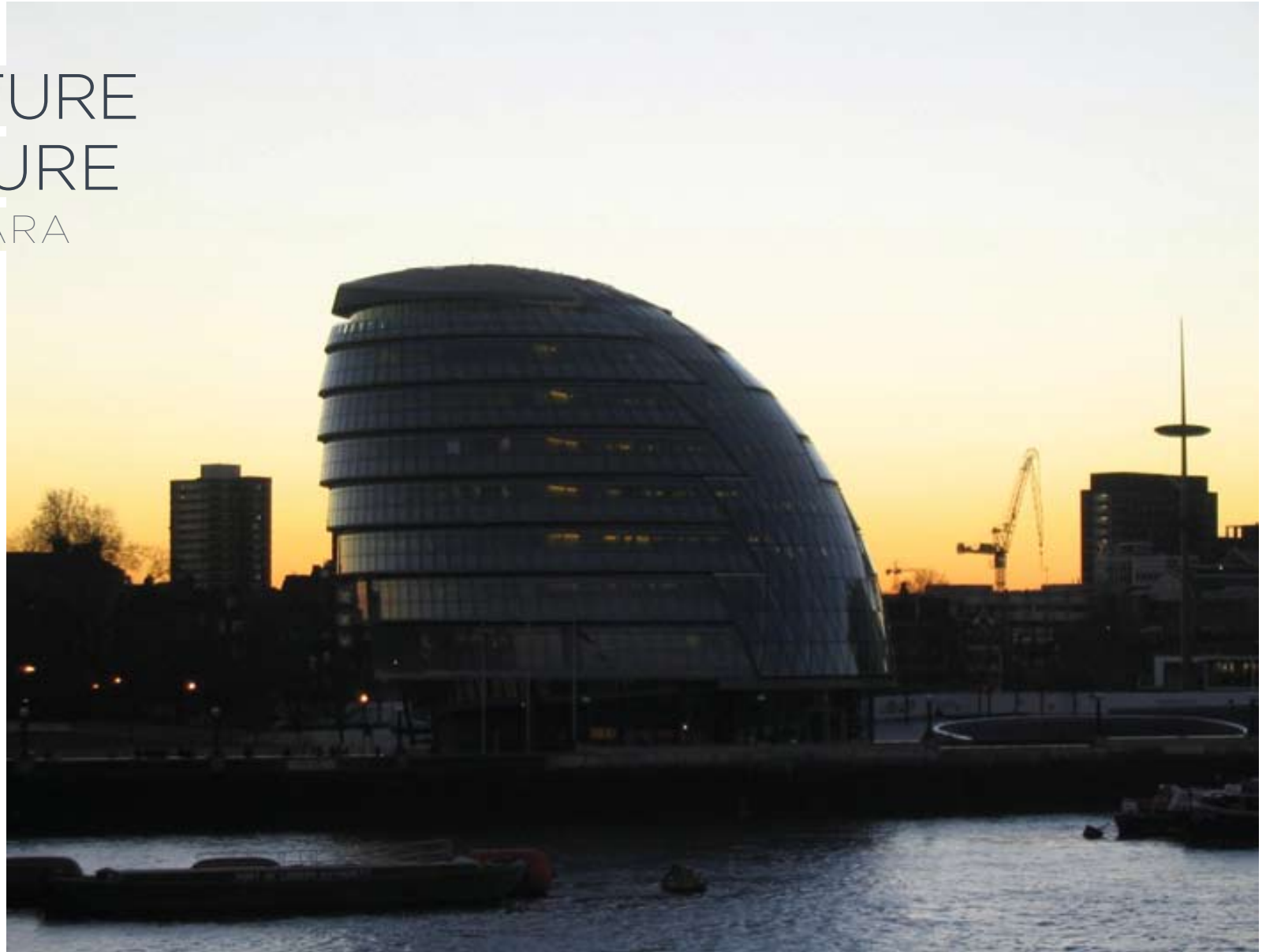
Above: View of the GLA building. (Image courtesy of the author).
